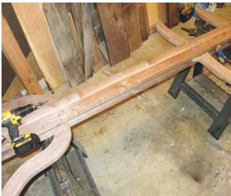
PIC 14. Pre-drilling and counter-boring screw holes for additional support
