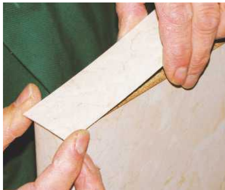
STEP 8. Allow the glue to dry, then position the lipping on the worktop, checking you've left an even overlap on either side
