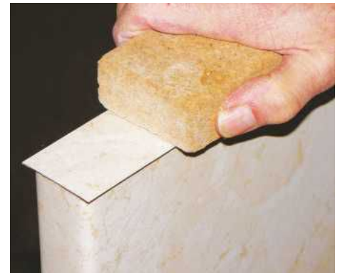
STEP 9. Next, use a cork sanding block or padded wooden block to apply even pressure to the length of the lipping
