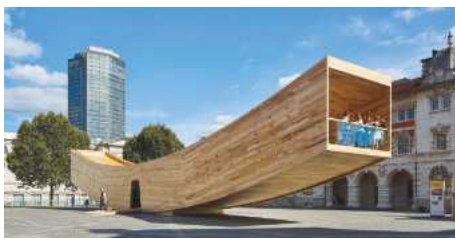
Conceived as a habitable arc and shortlisted within the Buildings Competition's 'Small Projects' category, The Smile was a 3.5m high, 4.5m wide and 34m long curved timber tube that cantilevered 12m in two directions with viewing platforms at both ends
