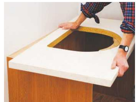
STEP 12. Replace the worktop above the unit and check that it fits snugly against the wall
