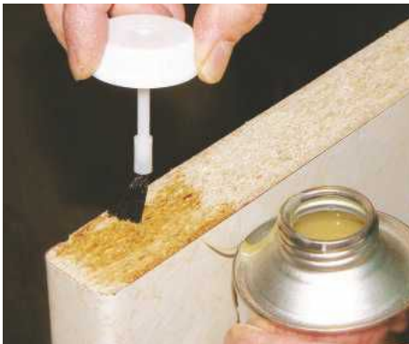
STEP 7. Brush contact glue along the worktop's sawn end, and the back of the laminate lipping
