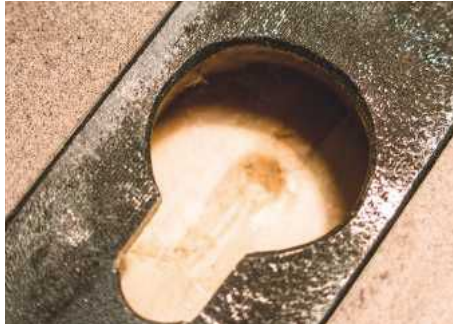
PIC 4. The keyholes were sized to accommodate 10mm self-tapping masonry bolts allowing only a couple of mil' play around the shank
