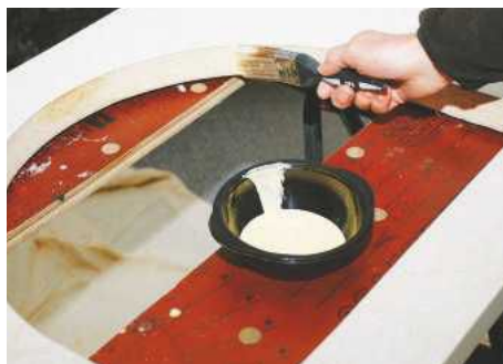
STEP 5. Brush PVA glue on to all sawn edges to seal against water penetration; alternatively, you can use silicone if you prefer
