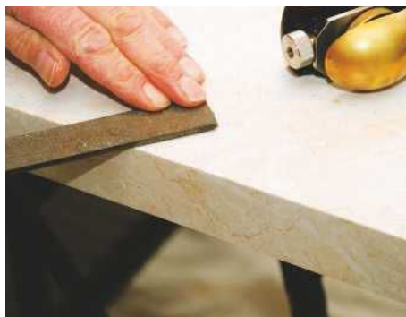
STEP 11. Use a second-cut file, titled, to smooth the lipping flush with the worktop surface
