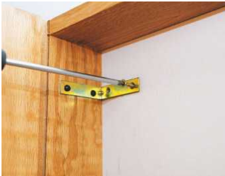
STEP 1. Start by positioning the cupboard base unit and fixing it firmly to the wall using steel brackets or similar hardware
