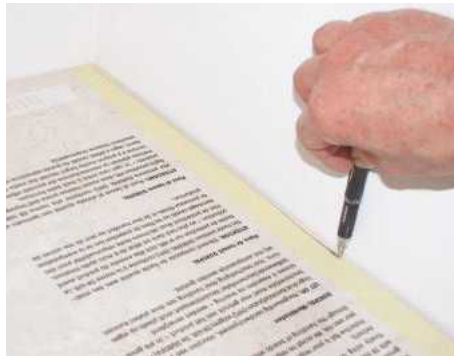
STEP 2. Place the worktop on the unit and run a pen against the wall for scribing with a jigsaw
