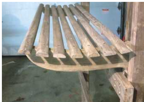
PIC 27. Slats screwed in place
