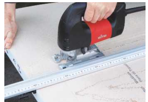
STEP 6. Saw the worktop upside down if you're cutting with a normal jigsaw blade, supporting the waste piece
