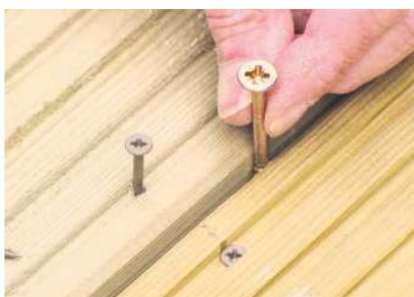
STEP 14. Boards should be fitted with expansion gaps of about 5mm; screws make ideal spacers
