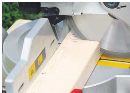
STEP 6. The next step is to cut all the short joists to exactly the same length, either with a mitre saw or by hand
