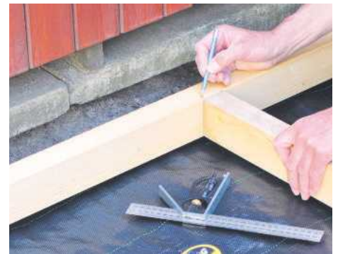
STEP 5. Mark out the positions of butt joints on the framework. Ideally, joists should be no more than 500mm apart
