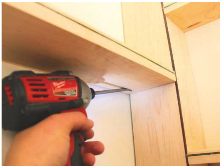
PIC 38. Take one Kreg screw and drive it through the pocket hole and into the post
