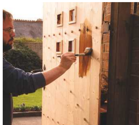
PIC 10. One of the most basic surface treatments is a water-based wood preserving stain
