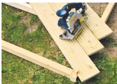
STEP 19. If you decide to fix boards diagonally, make sure you adapt the joist layout for adequate support
