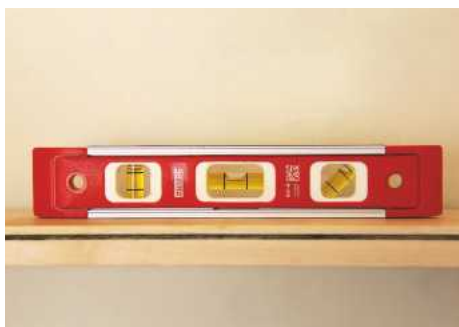
PIC 35. Check to make sure the shelf is level
