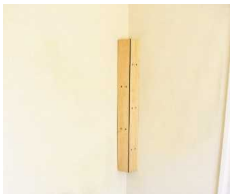
PIC 32. The corner post in position
