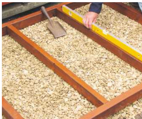
STEP 12. Check for level (front to back) and for sufficient fall across its length. Rearrange the gravel to increase height
