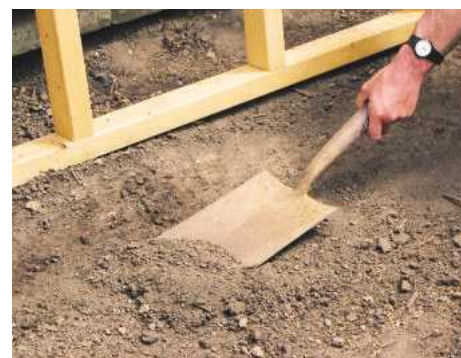
STEP 3. Flatten the area with a spade or shovel, though this does not have to be absolutely perfect
