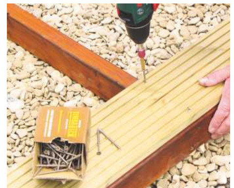
STEP 13. You can then screw the first board to the frame, keeping the leading edge flush if facing it with a vertical board later
