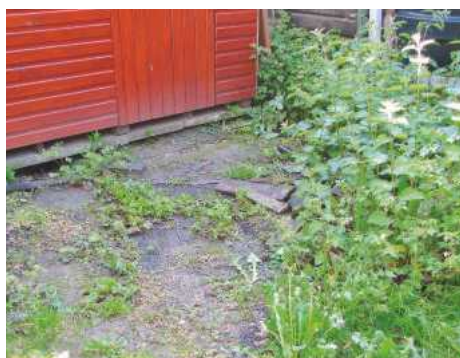
STEP 1. First clear the ground where the decking will be sited, using weedkiller if necessary
