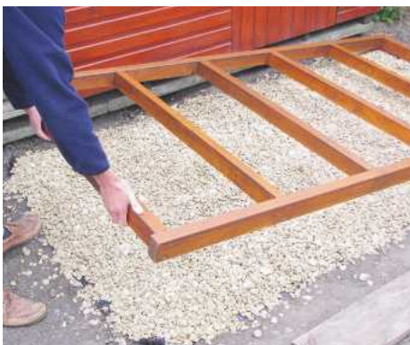
STEP 11. Lay the framework on top of the gravel and make sure it beds down reasonably firmly
