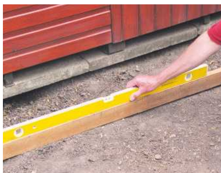
STEP 2. Check the ground for bumps and hollows, using a timber straightedge with a spirit level
