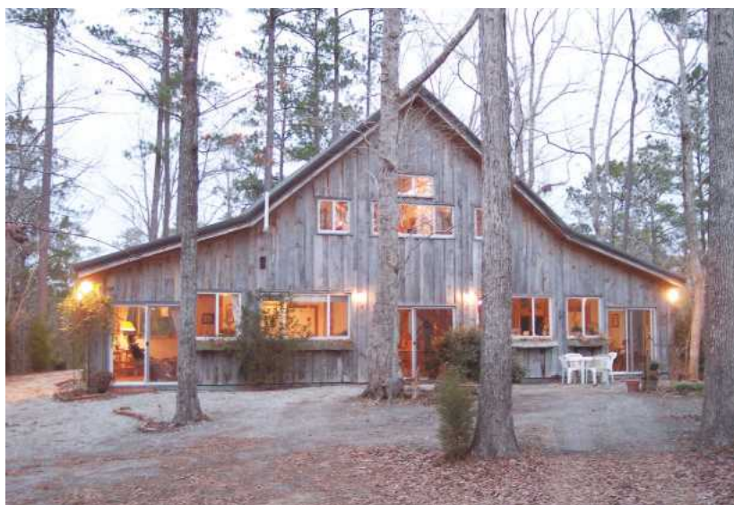
ABOVE: The exterior of Michael's stunning house, which he made himself using traditional methods
