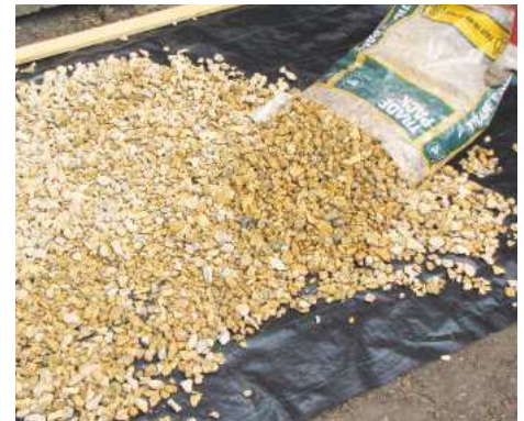
STEP 10. Spread gravel across the fabric to provide a bed for the frame and to soak up moisture
