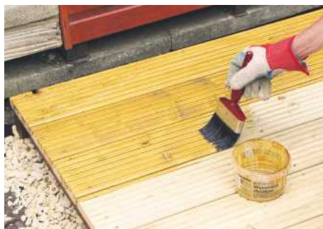
STEP 17. Increase the lifespan of boards by treating them with two or three coats of a suitable decking stain or oil
