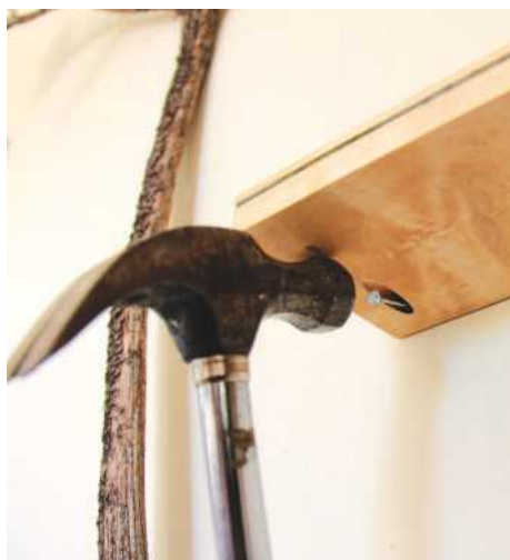
PIC 36. Use a hammer and nail to mark a point on the wall
