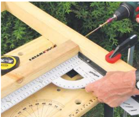
STEP 8. Cramp and screw through front and rear bearers into the cross joists, checking for square
