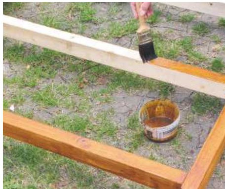
STEP 9. Once the framework is complete, brush on exterior stain to give the timber maximum protection
