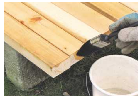
STEP 7. Timber may be pressure treated, but brush preservative onto all sawn ends of joists
