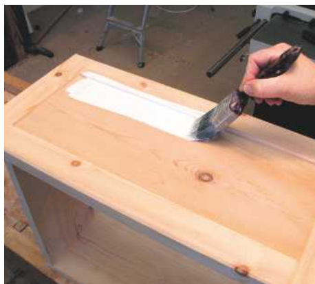
PIC 9. Primer paint applied to bare wood soaks into the surface and provides a firm key for later coats
