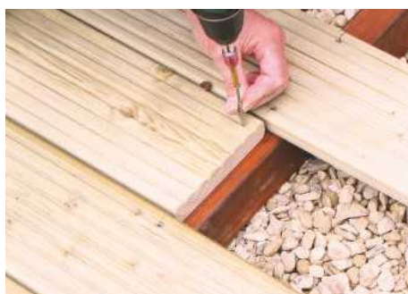
STEP 15. If you need to butt board ends together, stagger the joints across the bearers
