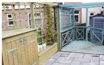
The original area ready for work (I thought it looked OK!)
