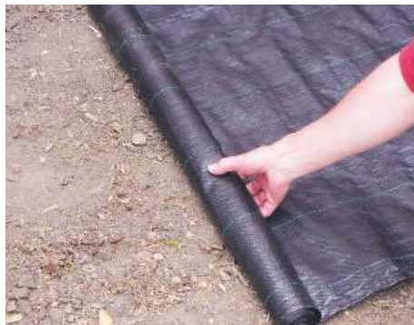
STEP 4. Once the soil is level, lay down heavy landscape fabric to prevent weeds coming through
