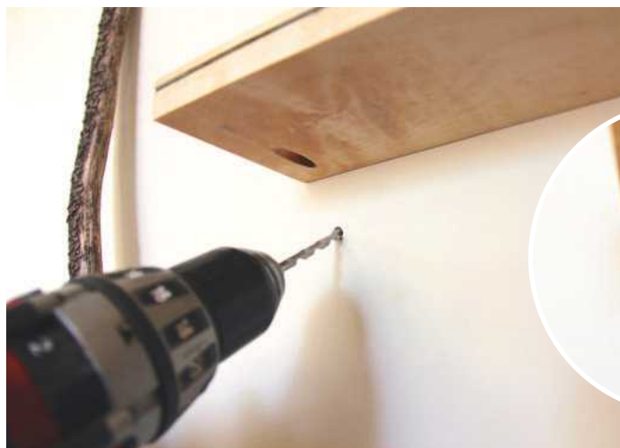
PIC 37. Remove the shelf and drill a hole into the plaster wall to fit the plastic anchor
