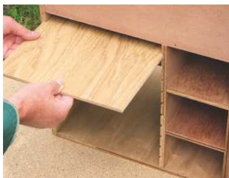
STEP 20. Cut sliding trays to size and check that they slide in the grooves. Add a finger hole if you so wish
