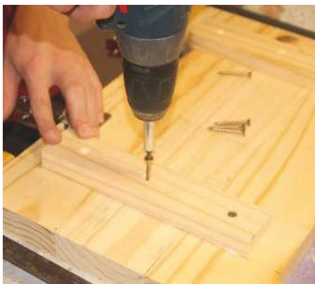
STEP 14. For added strength, a couple of supports can be added to the lid for the large step. These are scrap 22 x 44mm pine strips glued and screwed with 40mm screws
