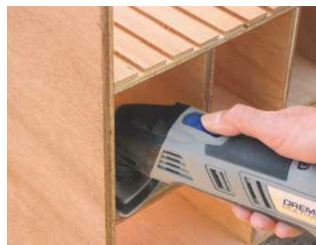
STEP 21. Fill any dents and clean up inner surfaces of the box with a detail sander, if necessary
