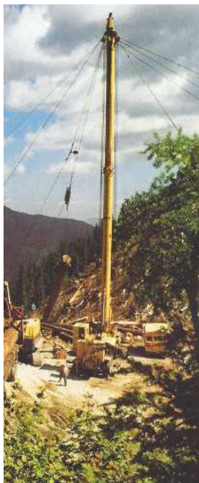
PIC 5. Using a steel cabling system to extract timber
