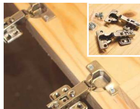
STEP 13. Secure the concealed hinges onto the top using 16mm screws
