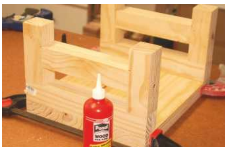
STEP 6. For the small step stool, glue the legs to the slat seat
