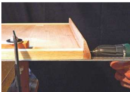
PIC 15. Drilling to attach the bookrest
