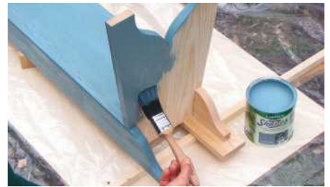
STEP 27. Brush on at least two coats of suitable paint or clear varnish. Replace hinges when fully dry
