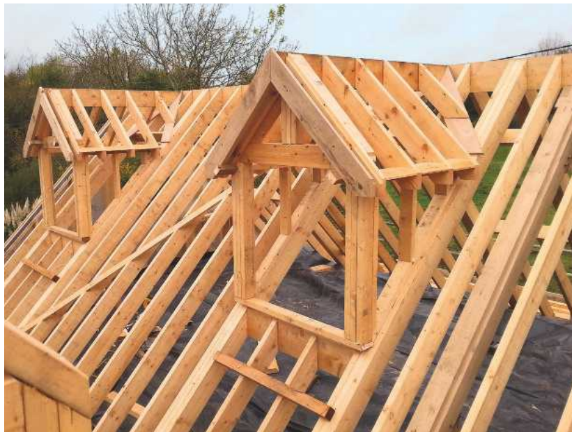
ABOVE: A roof under construction
