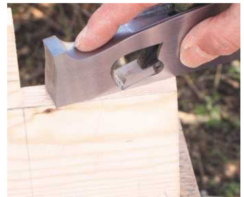
STEP 7. Clean up the sawn notches with a shoulder plane or chisel and check for square
