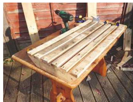
PIC 9. To finish the top shelf, I added another piece of wood underneath, for increased stability
