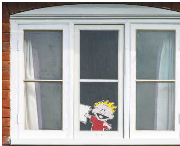
ABOVE: One I made earlier: a plywood blank protects a window opening against the weather and takes the jeopardy out of removing casements, sashes, or entire frames and leaving the house open to the weather; a trompe l'oeil is optional
