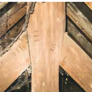
ABOVE: Hand-made: a joiner's marks pair up the mortises and tenons of a king post and its struts in The Old Vic's roof
