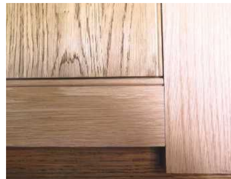
PIC 13. Detail showing hand and machine-made corner beads
