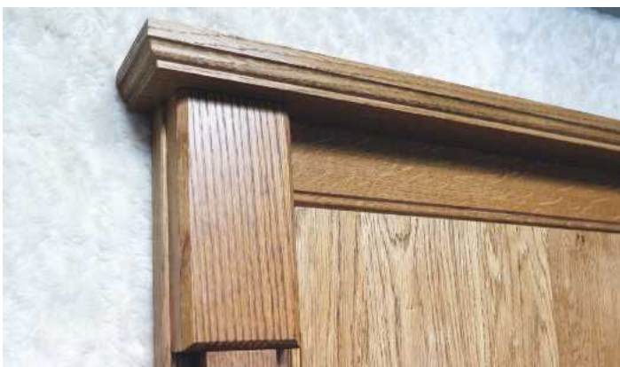
PIC 16. Top of board showing block and coving
