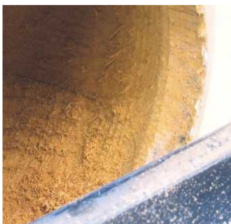
STEP 13. The finish left on this dry oak is not perfect but you can remove timber really quickly. It is best to clean up the surface with a different tool when most of the waste is removed
