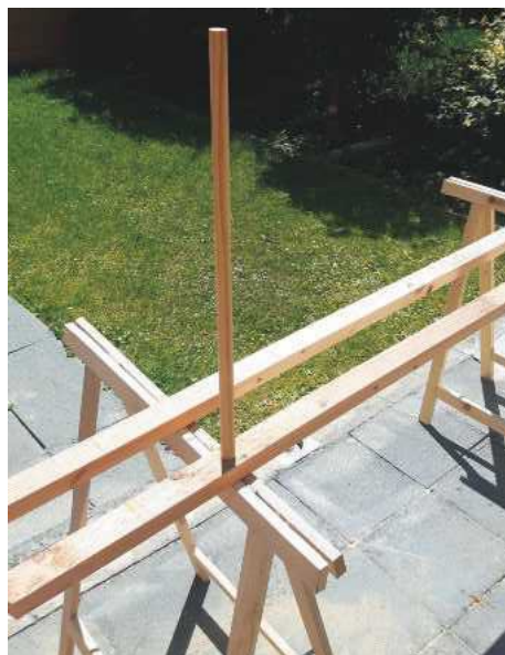
STEP 4. Test one of the safety gate spindles in the hole before drilling the remaining holes
