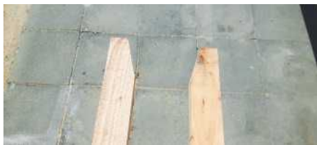
STEP 2. The tops of the ladder – these need to be test fitted to ensure they fit nicely to the wall
