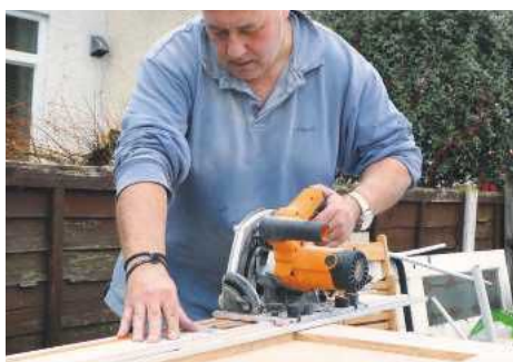
The saw left a very clean finish when cross-cutting this oak door to length
