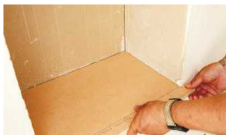
The resulting fit will be tight and clean on all edges
