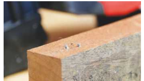
You can adjust the drive to suit the timber. In hardwood it needs a higher setting to drive fully
