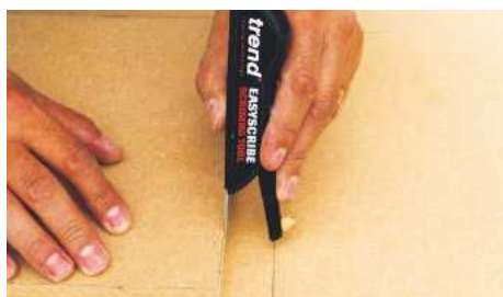
Keeping the same setting on the EasyScribe, transfer to the cill board and cut to the marks
