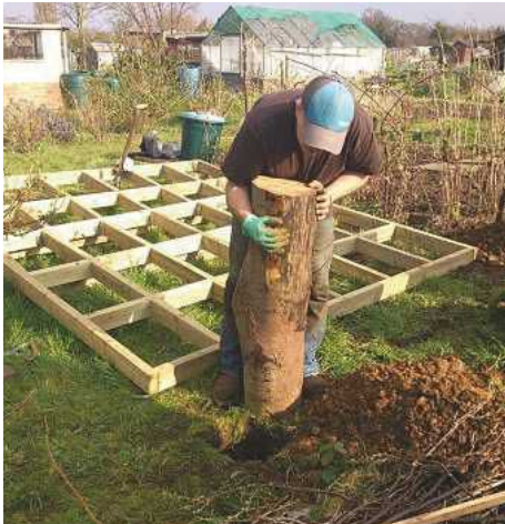
PIC 1. Sinking the log foundation posts
