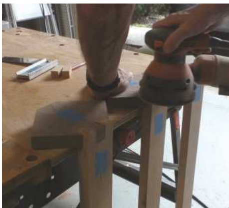
STEP 25. After the glue sets, the joints need to be sanded smooth
