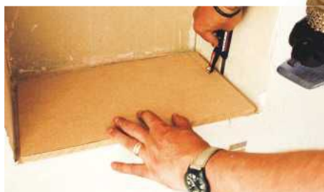
You can spile by opening up the EasyScribe and marking around a template board
