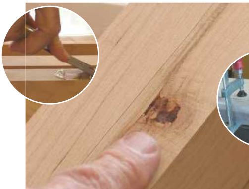
STEP 7. Filling the voids with clear epoxy helps to give the wood character, although this is optional
