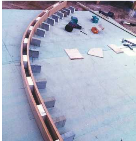
PIC 2. Each rib was curved along a former
