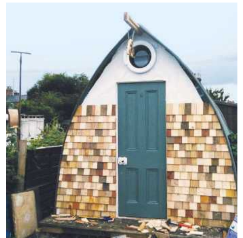
PIC 6. The lengthy task of fitting the individual hardwood shingles
