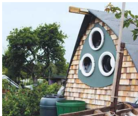
PIC 8. Washing machine doors were repurposed as windows
