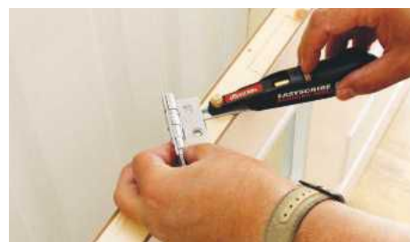
A thicker hinge can be marked up for leaf thickness using the EasyScribe
