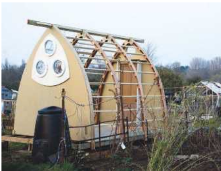
PIC 4. The frame erected on the plot
