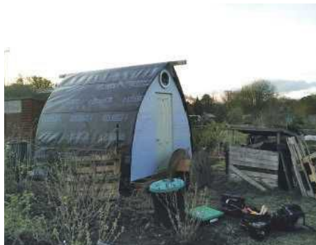
PIC 5. Roof skinned and waterproofed
