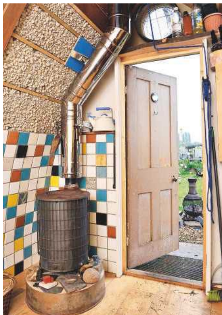
PIC 7. The stove was fitted using brand-new double-walled flue, to make it as safe as possible
