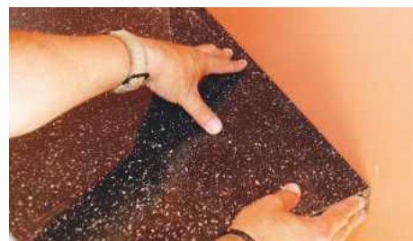
Planed to the line, the fit is perfect
