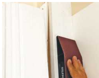
Cutting back filler was very quick and you can sand right up to an edge
