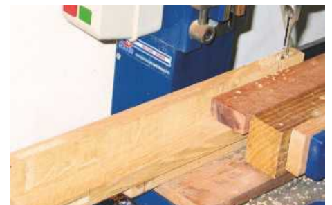
STEP 9. Pack out and chop the mortise holes
