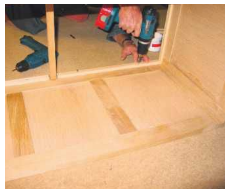
STEP 17. A few softwood battens are fixed in place to take the bottom
