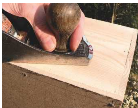
STEP 16. Trim the MDF edges flush with the sides of the box and make sure all nail heads are flush
