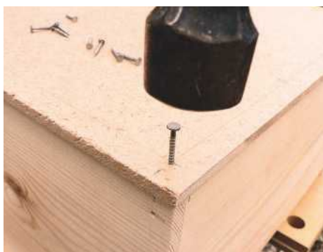
STEP 15. Cut a piece of 6mm MDF slightly oversize for the back. Glue and tack to the carcass with 20mm ring shank nails
