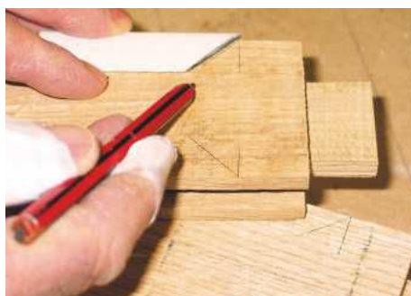
STEP 13. A plastic template can be used to mark out the ends of the bevells
