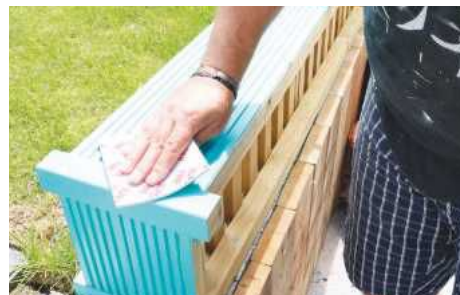
The base coat is de-nibbed with a fine abrasive and dusted off
