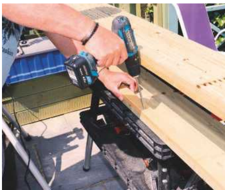
STEP 13. Battens are screwed inside at the bottom, ready for the base
