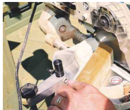
STEP 4. Setting the mitre saw to 30°, cut a mitre and then rotate the leg
