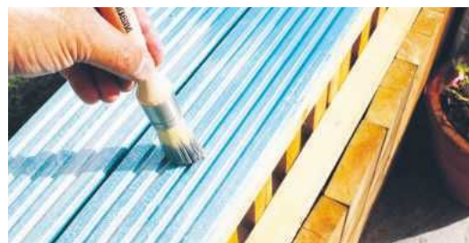
As you brush it in the silvering becomes apparent while the blue still shows through
