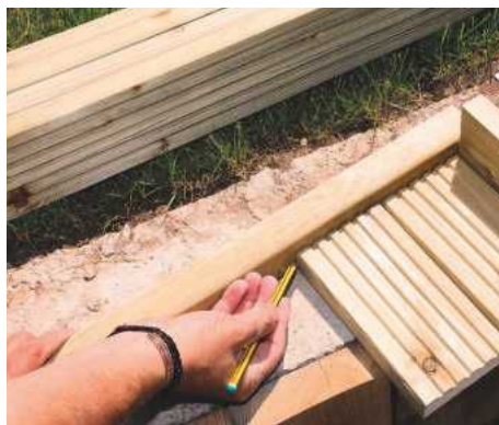
STEP 3. Using deck boards as gauge blocks, mark the legs to length and cut to size
