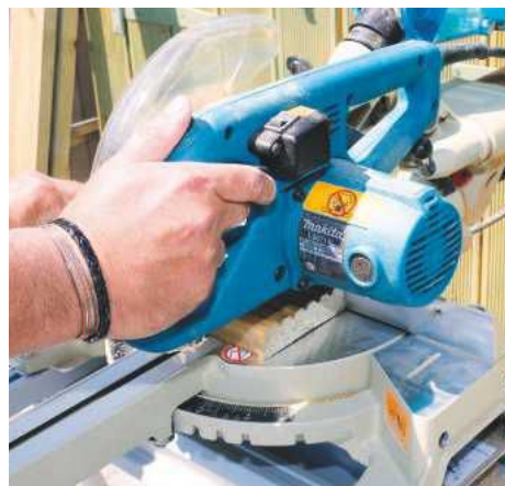
STEP 2. Cut all the deck boards to length using the mitre saw, or by hand if you don't have one
