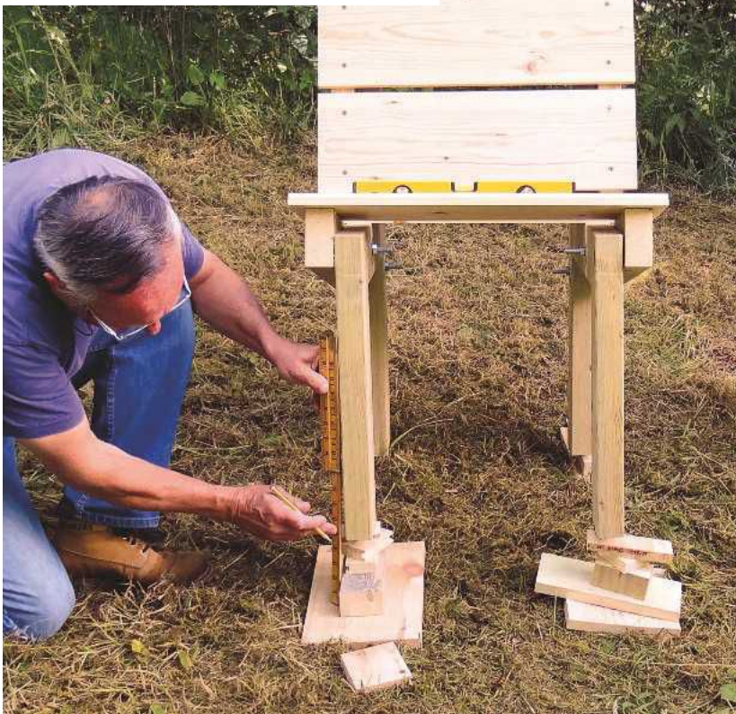
PIC 8. I've scribed units into walls before, but I've never scribed a chair into a hill. I might have levelled the ground instead, but to do so would, in my mind, impinge too heavily on the landscape: I want to tread more lightly. Initially the chair back was one plank higher but that really was superfluous. I hadn't realised until I put the chair in place that a front fascia would be needed to balance out the chair's visual weight
