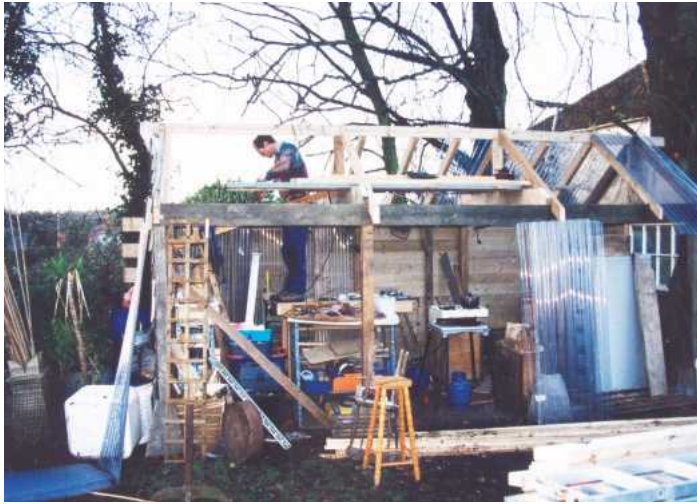
PIC 1. Getting the first rafters and the ridge set up is always the difficult part if working on your own
