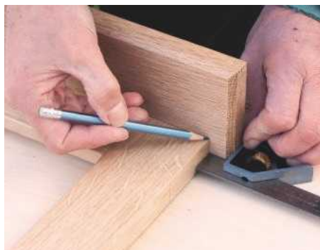
STEP 15. Mark the position of the shelf. This can either be pocket-screwed or biscuited to the frame
