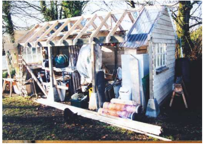
PIC 2. The end of the day with a range of rafters all in place
