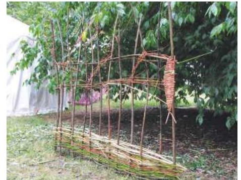
A willow fence partly built
