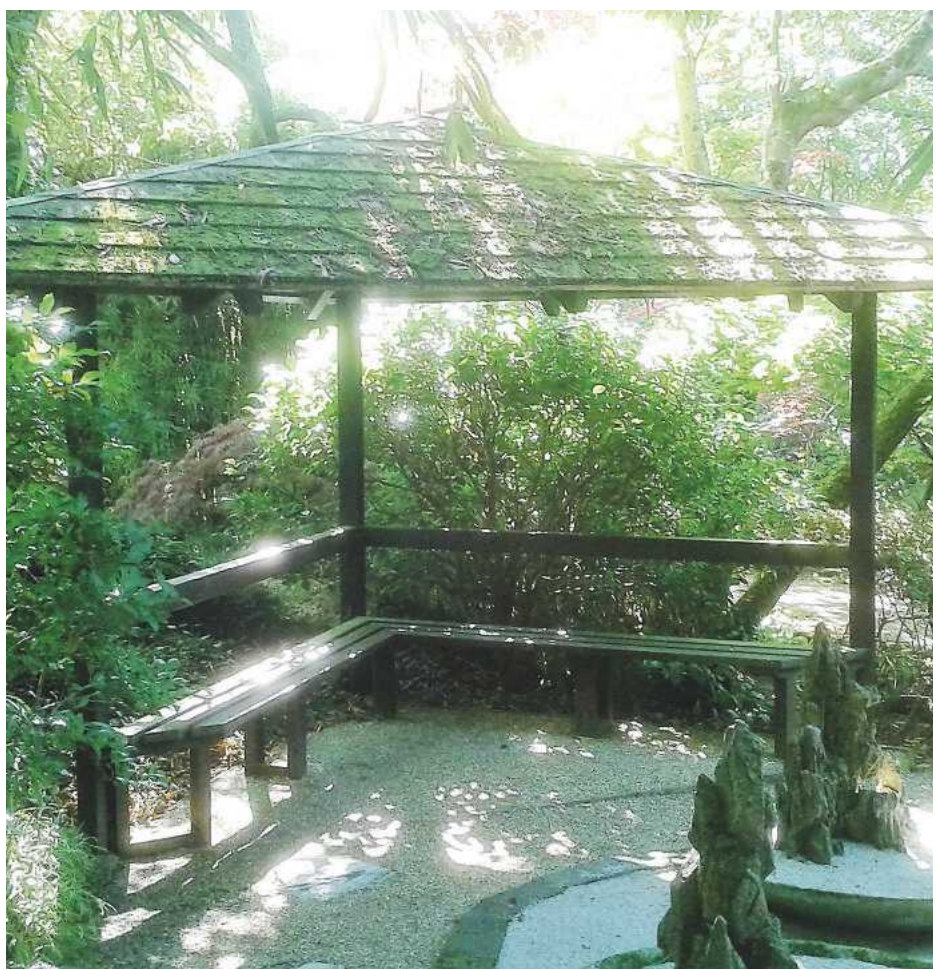
PIC 12. A simple Japanese-style garden shelter. This is challenging because the whole thing is held up on three posts
