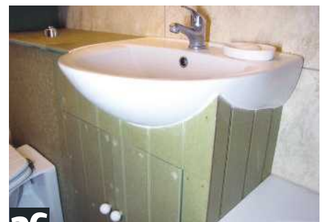
36 Using a cartridge gun, apply a bead of silicone sealant around the basin. Smooth this off while it's still wet
