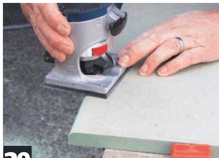
29 Cut an 18mm horizontal panel to sit above the cistern. Rout the front edge with a bearing-guided roundover bit
