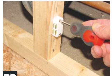
33 The 6mm bath panel is light enough to be attached with magnetic catches. Screw sufficient blocks to the framework
