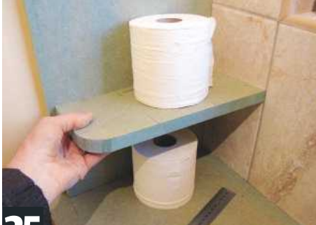
25 Scribe and cut an 18mm panel to the end wall. Temporarily screw this in position, then mark out suitable spacings for each shelf
