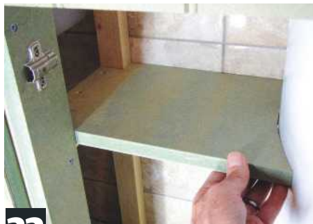
32 Add a shelf inside the cupboard if there's space. Making an accurate card template first will ensure a neat fit
