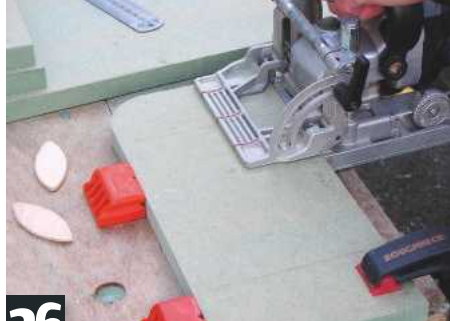
26 Shelves are fitted to the wall panel with No.20 biscuits. Mark out and cut slots with a biscuit joiner
