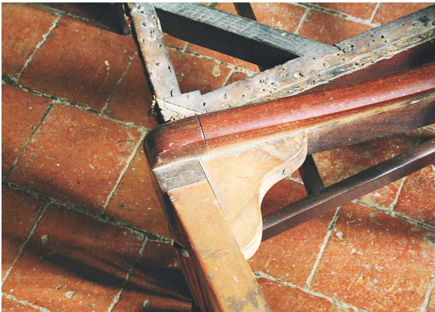
Here are some 18th- and 19th-century chair braces. The former is unusual in that it's at the front rather than the back
