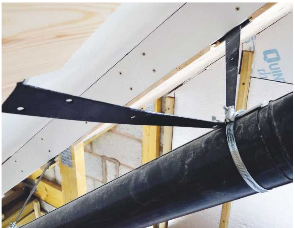
These standard Japanned 'T' hinges were ideal for holding the flue pipe in place
