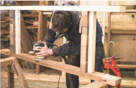
Cleaning up one of the hollow cupboard sections; the timber frame is just for temporary support
