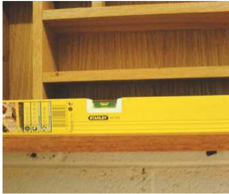
▲ Pic.21 Once the other cleat has been attached, lift the cabinet onto the wall
