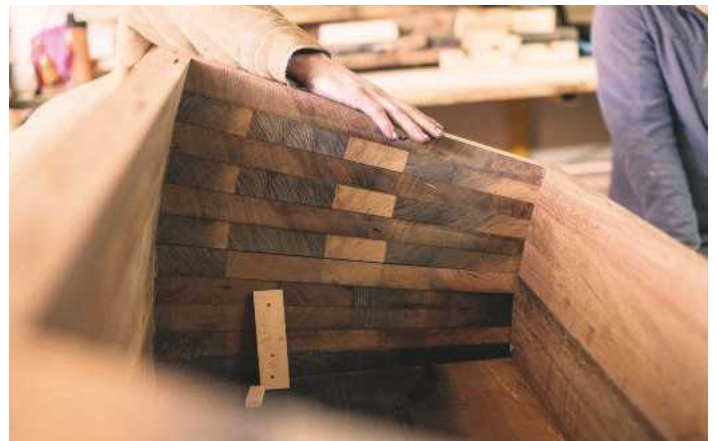
Pre-assembly checks ensure that all will be fine when it comes to the final glue-up
