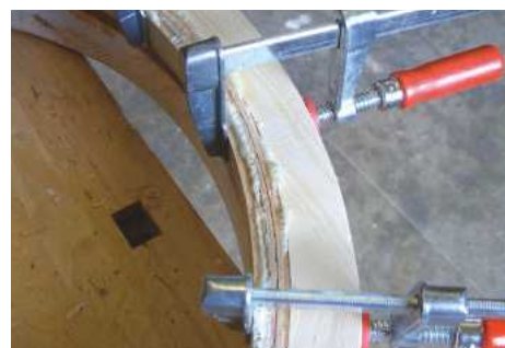
▲ Pic.12 Glazing strips are laminated from 2mm thick oak strips, glued together inside the frame
