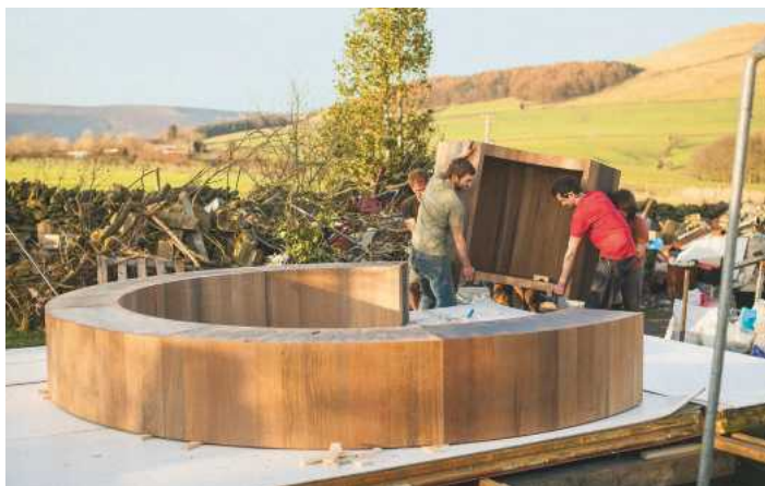
Putting the pieces together in a dry-run installation – fingers crossed the reality matches the drawing
