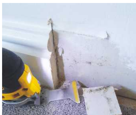
▲ The resulting finish is clean and smooth
