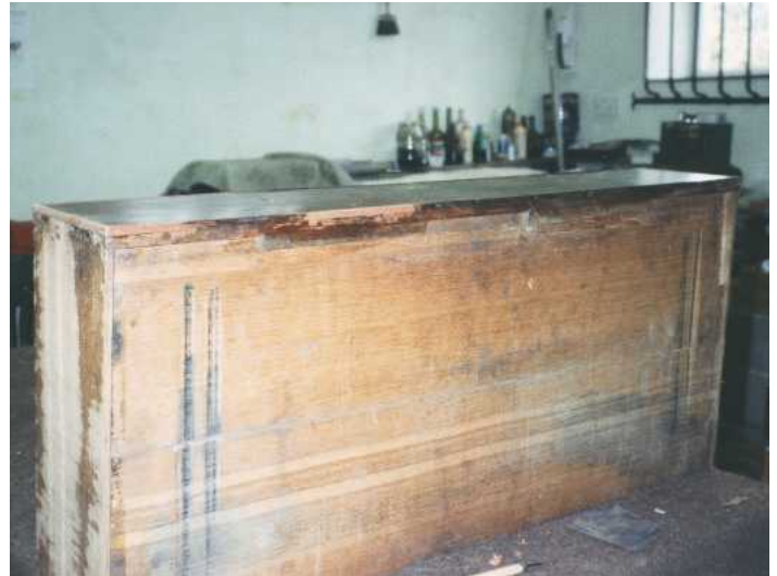
▲ Pic.7 45° for security: new sections of beading are better fitted with a scarf rather than just butted; corners are mitred
