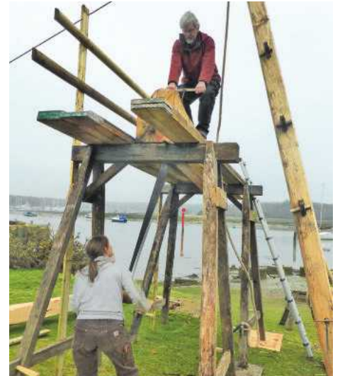
Pic.4 Once hewn, the logs can be sawn into smaller timbers if required. Traditionally this was done either over a pit or on trestles as here. The hewn log is lifted up using the timber crane
