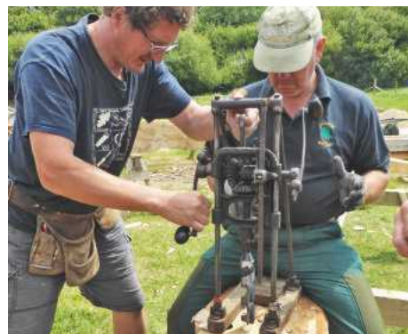
Pic.7 John, Henry's twin brother, is carefully positioning the boring machine, before the seated student will auger part of the timber away that separates the wallplate tenon from the second tenon. Then the back cheek of the wallplate tenon can be pared back to its lines. The second tenon will fit into a tie beam that lies above the wallplate
