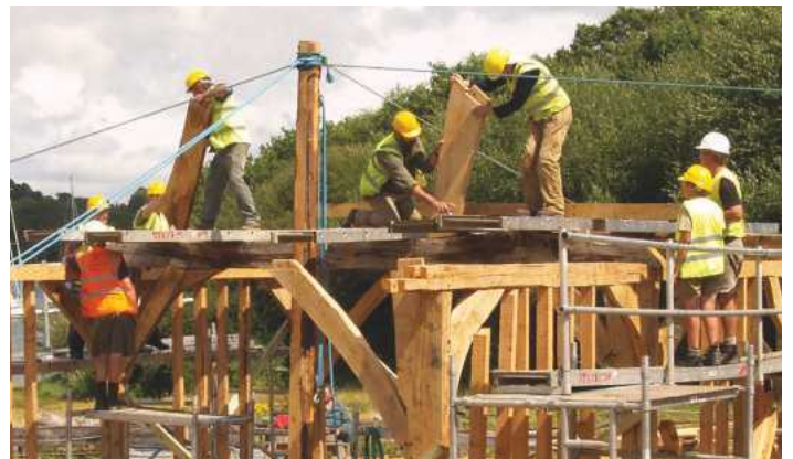
Pic.18 The gin pole has been moved and behind it a queen strut is man-handled up
