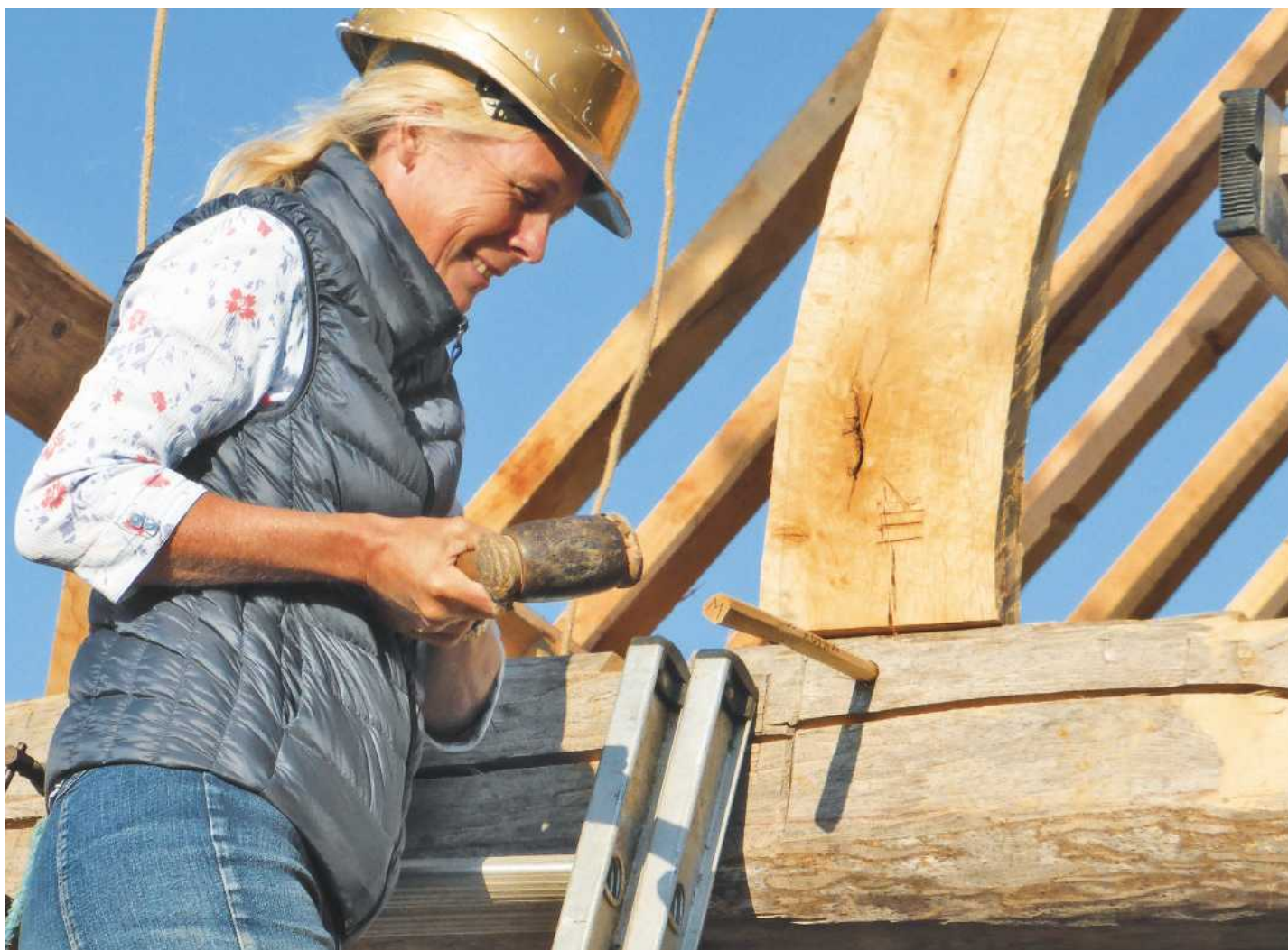
Mary Montagu-Scott knocks in the last peg; inset, the almost finished building
