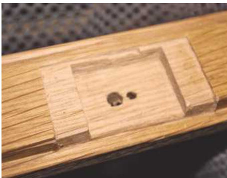
▲ Pic.32 Drill holes in the door frame, then connect the holes to create the keyhole
