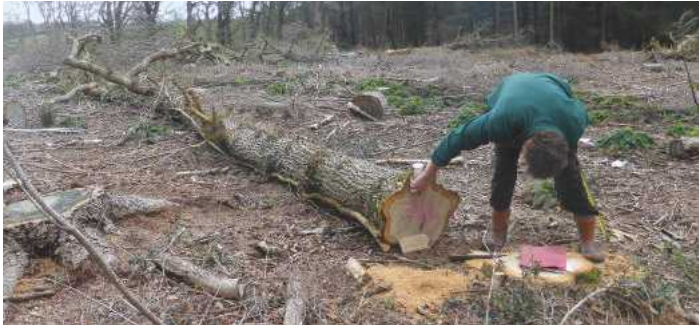
Pic.1 The timbers were felled locally and Master Framer Henry Russell selected which logs were to be used for each location. The oak was chosen standing and with a view to which component it would provide – in this case a tie beam. However it is only when the log is felled and converted that you actually know what size you will get
