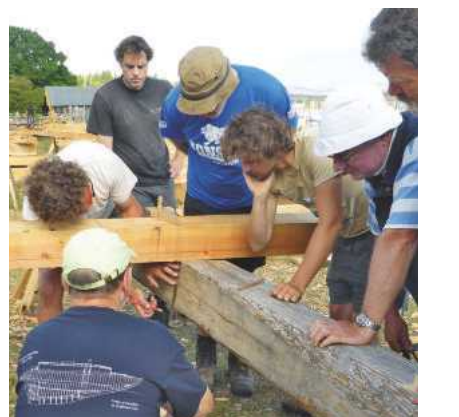
Pic.10 Henry Russell demonstrating the use of the plumb-bob to scribe two irregular timbers together. Note the 'doughnut' shape of the plumb-bob that also allows it to be used over a full-size drawing of the building, if required. Precise, careful lining out is essential for successful timber framing
