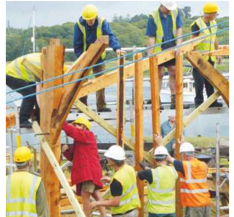
Pic.14 Wiggling the next heavy tie beam in between the existing studs was interesting!
