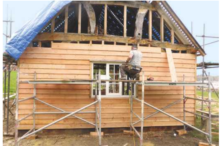
Pic.29 External cladding and windows now going in
