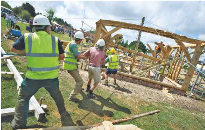
Pic.17 ...and locating all the studs as it is lowered. You can see them looking to locate the tenons on the underside – a fiddly and finger-crushing job!
