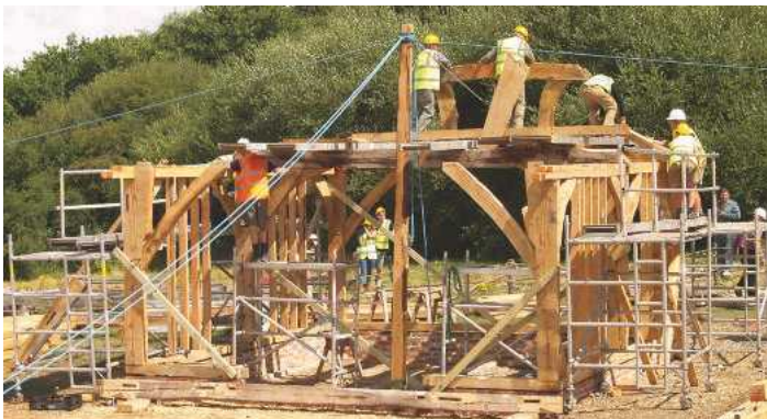
Pic.19 The roof collars starting to be built up
