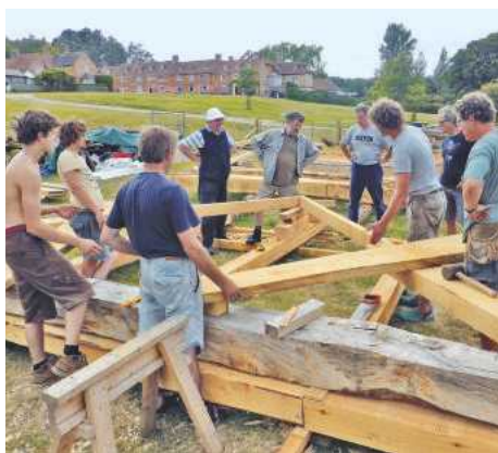
Pic.9 Because the timbers are not square, the best way of laying out the joints is to set up each roof truss assembly on a dead flat surface and scribe the joints. Here a cross-frame roof truss is laid out before scribing. The tie beam (large timber in the foreground) will have a pair of diminished principle rafters tenoned into each end of it. These will be stiffened by the pair of raking struts or raking queen posts (the diagonal timbers in the middle). The students pay close attention to the master's words!
