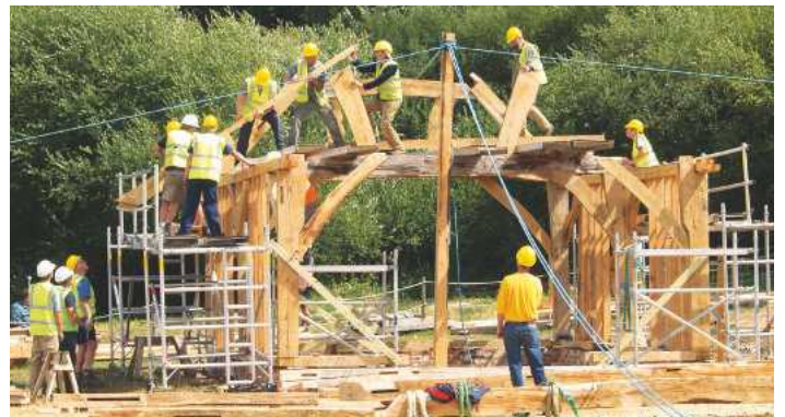
Pic.20 A diminished principle rafter going in
