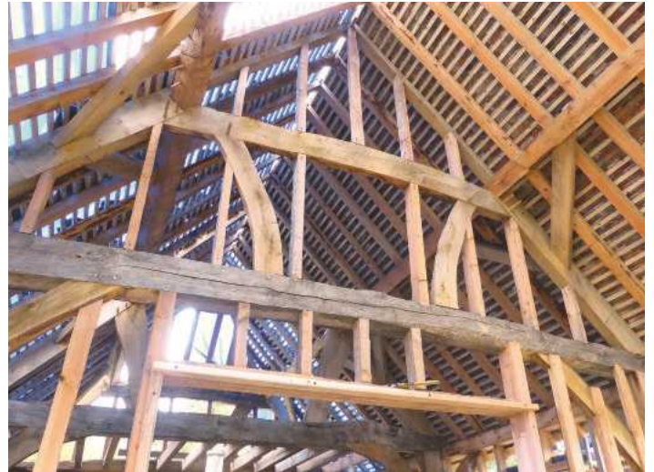
Pic.28 A view of the bay structures, showing clearly how the roof is supported
