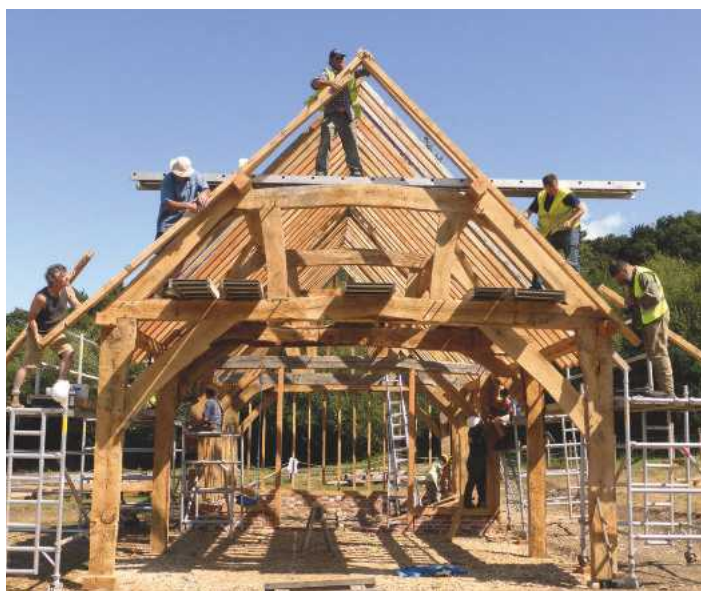
Pic.25 Common rafters being fitted before the last peg is knocked in
