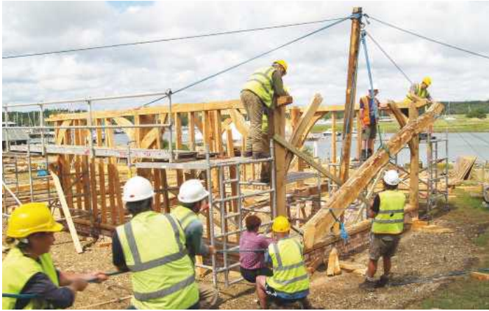
Pic.13 The first tie beam being hauled up using a 'gin pole' crane. The pole can be moved around easily for each big timber as the roof is erected
