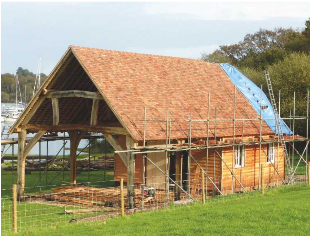
Pic.30 The roof almost complete – note the covered open bay, a feature often forgotten when workshops are designed
