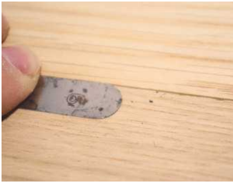
▲ Pic.7 ...the aim being to finish with the frame very slightly proud of the MDF
