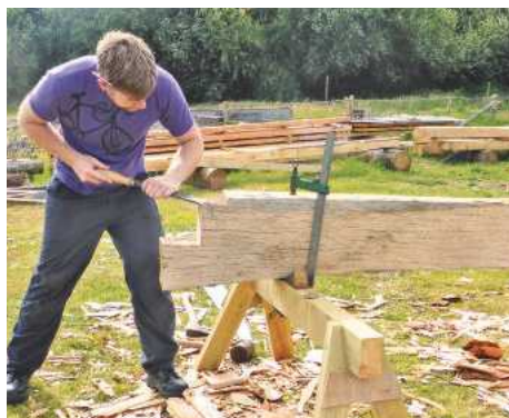
Pic.6 Tenons are often cut with a saw and chisel. Here the front cheek of the wallplate tenon, at the top of a jowl post, is being pared down to the line. A second tenon will be cut, later on, out of the swelling or jowl, below this wallplate tenon. In all construction the joint itself has to be cut no deeper than the minimum cross-section of the timber required to resist bending and twisting and shearing forces
