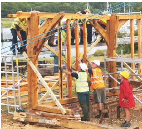
Pic.17 ...and locating all the studs as it is lowered. You can see them looking to locate the tenons on the underside – a fiddly and finger-crushing job!
