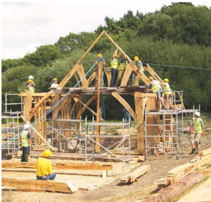
Pic.21 Now the roof structure can begin to be seen
