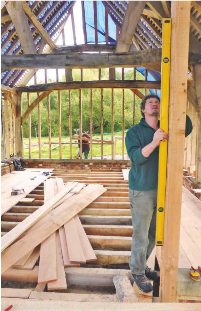
Pic.27 Internal fitting-out beginning
