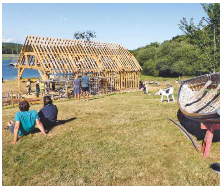
Pic.26 The frame finished and waiting for roof tiles and cladding
