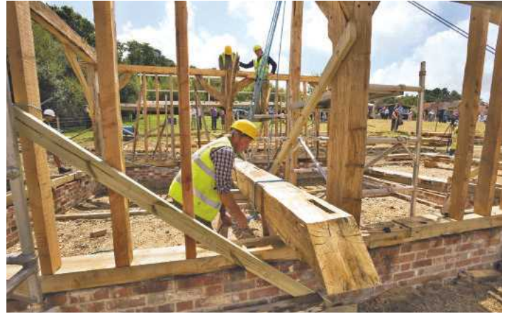
Pic.14 Wiggling the next heavy tie beam in between the existing studs was interesting!
