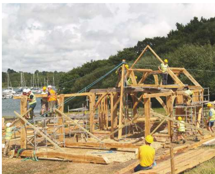
Pic.23 The open bay at the front is starting to be assembled
