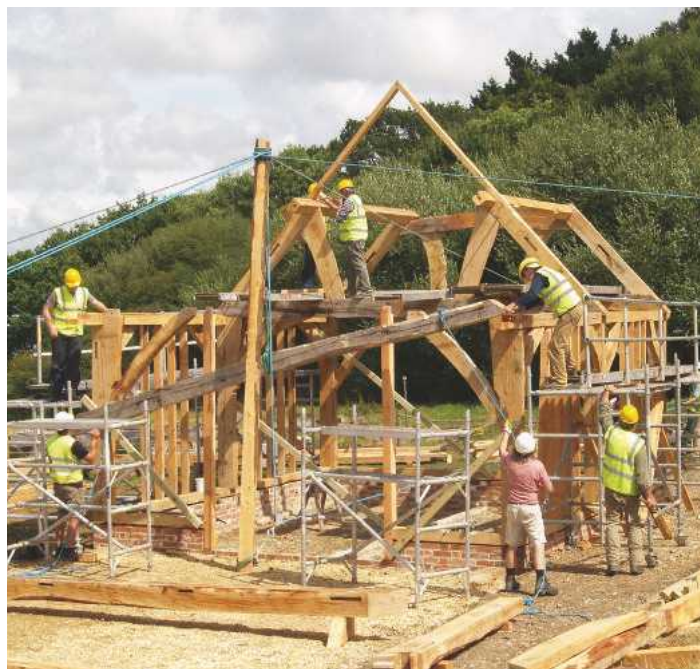
Pic.22 The last tie beam going in
