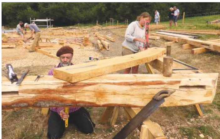
Pic.11 Andy and Barbara carefully laying out a brace, prior to scribing. The brace will tenon into the tie beam and jowl post. In the background others are cutting joints
