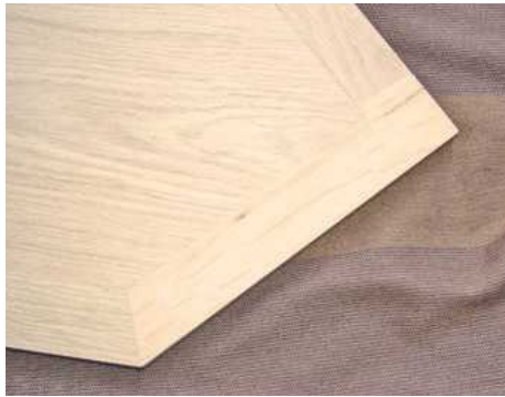
▲ Pic.8 Rebating prior to jointing would've been easier, but the finished effect is not too unsightly
