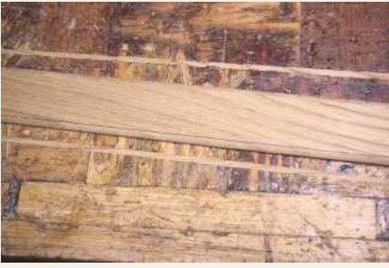
▲ Pic.1 Plane the top face of strips of oak until the thickness is 8mm. This will be achieved when the plane blade just breaks into the small rebate above the bead, and a very thin sliver peels away
