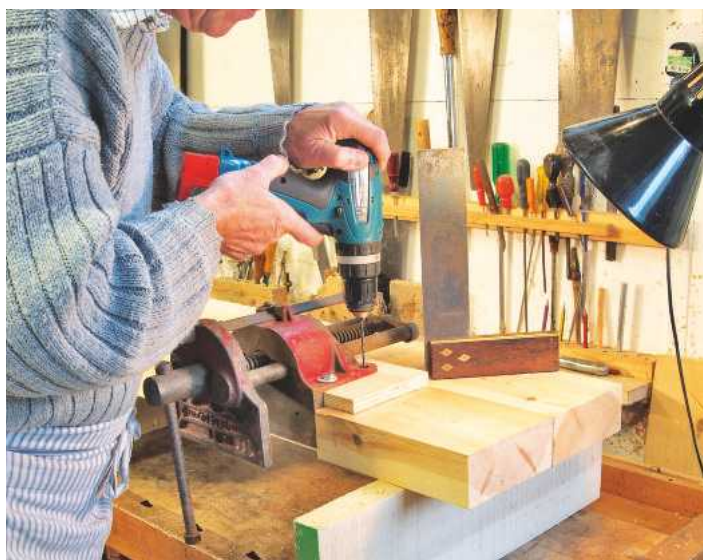
Pic.10 Drilling the marking holes for the counterbores
