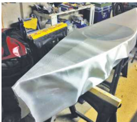
Pic.14 Glass cloth draped over deck
