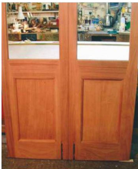
▲ Pic.7 The inner face of the doors; the ovolo moulding is a replica of mouldings on the existing shutters
