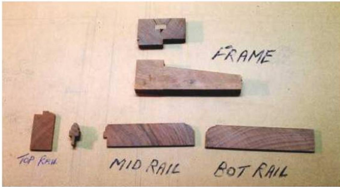
▲ Pic.1 Joinery section used as reference when marking up
