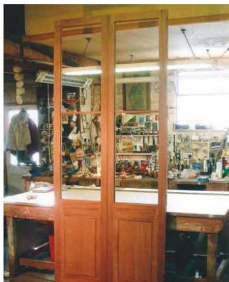
▲ Pic.8 The outward face of the doors; the panels are flush, surrounded by a captive bead – typical of mid-Georgian work
