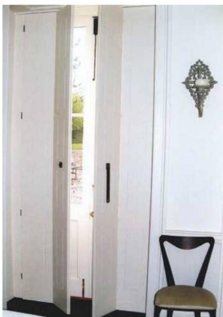
▲ Pic.10 The shutters are being folded into the centre
