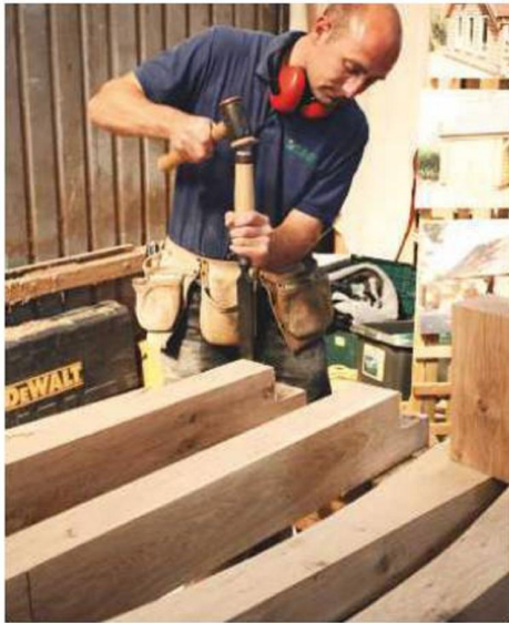
A Townsend timber man gets to work with the chisel...
