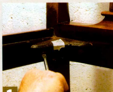
1 First label each part on masking tape before taking the joints to pieces
