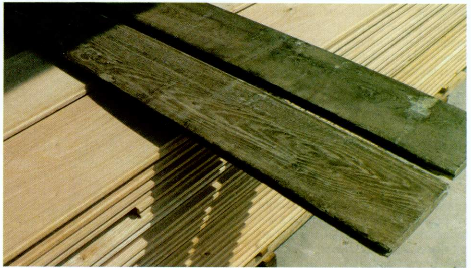
▲ These oak floorboards are actually new but have been aged to blend with period buildings
