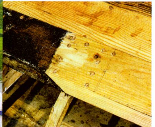
▲ A scarf joint on clinker planking, glued and copper rivetted as part of the restoration course
