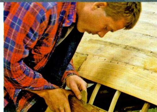
▲ Student Ira Jones sands back varnish on an old boat to clear lands ready for a new plank
