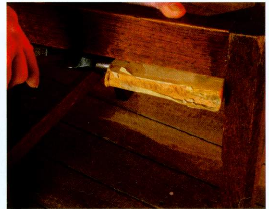
▲ Pic.2 Tapping may be enough to open the joint
