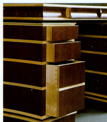
Drawer detail from the Parasol Desk, contrasting sycamore and purpleheart
