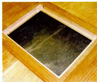
06 Alternatively, you might prefer a square insert, in which case rebate the relevant edges of the frame
