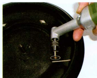
05 The fine crack was opened up using the Proxxon angle drill with a small blade mounted
