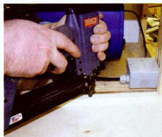
10 Now cut and pin a 15x15mm batten all round the inner edge to act as a stop for the inner filter
