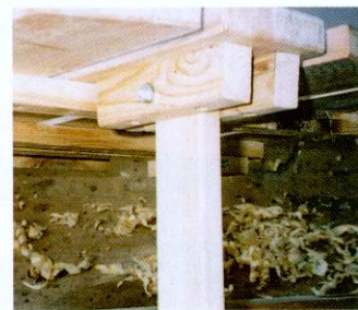
08 Additional short battens are added where the table legs meet the table top and bolt into place
