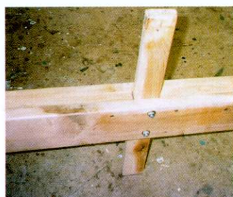
05 Then fill the gaps between the beams either side of the legs with lengths of 50x32mm timber
