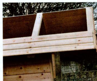
14 Work from the bottom up as you apply the shiplap. Don't forget to allow a slight drip overhang at the bottom
