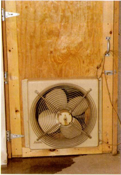
Immensely powerful, this window fan in the bottom of the door sucks most if not all of the airborne dust to the outside
