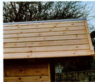
15 A strip of lead along the ridge will finish off the roof, making it neat and waterproof - within reason!
