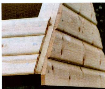
13 This is done on the ends of the roof timbers as well. Here one fillet will cover both exposed edges
