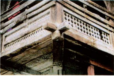
An example of cantilever construction to construct a veranda
