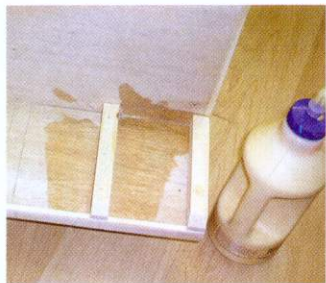
09 Space out the dividers on the side base extensions to accept a pair of Bessy clamps in each case
