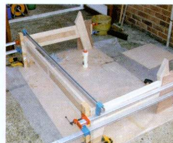
08 Sit the assembly on a perfectly flat surface as you assemble to ensure there are no twists in the finished frame
