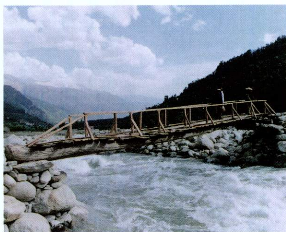
A single log bridge over one of the many raging mountain torrents. These bridges are easy to replace if washed away, which somehow you assume will happen regularly
