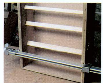
07 Cramp up, check for square, then set aside to dry before attaching to an appropriate wall
