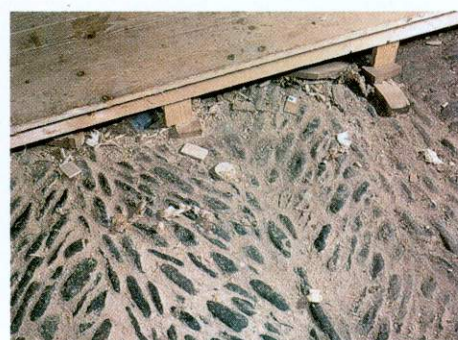
The original floor of the barn consists of pebbles from a nearby beach. Raised timber decking at one end makes it easier for Andrew to work
