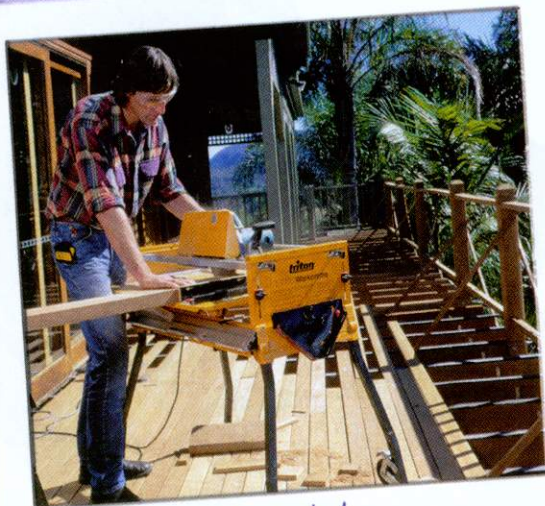
Gary building the rear deck
