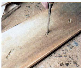
05 Drill out the mortices for the bars on a pillar drill to the correct depth then square up with a sharp chisel
