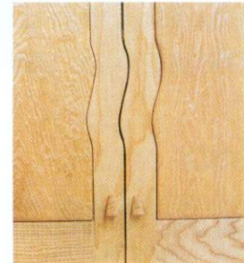
Door detail of an ash cabinet. The panels are rippled ash and contrast with the plainer rails and meeting stiles
