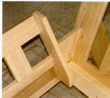
Bottom: Details of the rear arm rest cradle and the back rest supports
