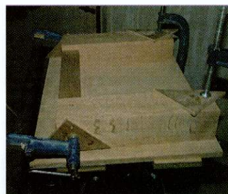
07 Assemble the end frames first and make sure they are square and out of twist. You may want to lime wax first
