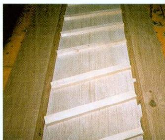
13 Simple 'go bars' apply spring pressure to the top mouldings. Mitre the ends neatly as you fit them
