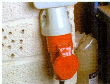
Three phase sockets are red, 16A ones blue and 110V ones yellow
