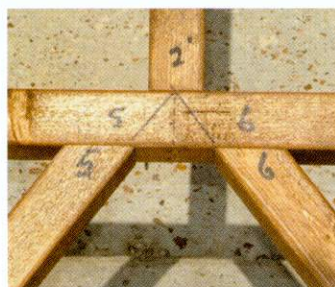
18 Mark off the dormer angles from the centre and cut diagonal trimmers to the correct angles and screw in place
