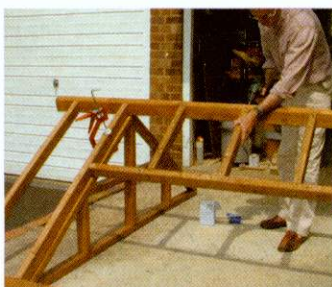
17 The front roof frame is trimmed as shown to accept the front dormer. This isn't essential but looks great
