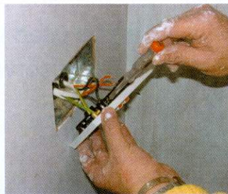
10 Make sure there are no exposed bare wires as you connect to the terminals. Sheath the earth wires
