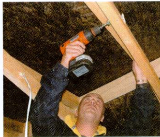
06 Drill the cables through studs and joists, ensuring the holes are large enough not to chafe them
