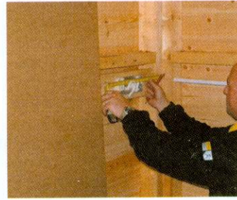
07 With the electrical carcasing complete, you can board out the workshop, cutting holes for pattresses
