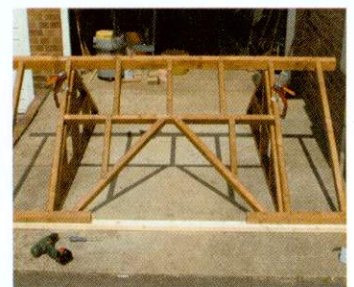
20 This is the front frame trimmed ready to take the dormer extension. James used the gable ends to support the frames
