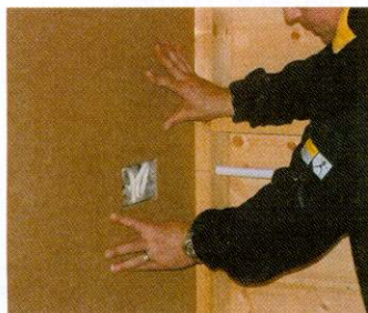
08 Measure or mark out the apertures carefully so that the back boxes sit neatly in them. Fix the boards in place
