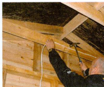
05 Even in the roof space keep the cable runs clipped back and tidy, and out of reach of errant nails
