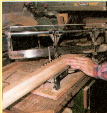
10 A mitre saw will be needed for a neat joint on the mouldings. Cut the front piece to length first then cut the sides to fit
