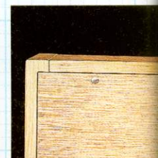
The back of the breadbin is rebated into sides and top
