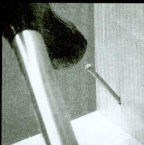
Carpenters spike the nail at an angle for butt jointing. In cabinet work it is best to pre-drill the first component otherwise the grain will split
