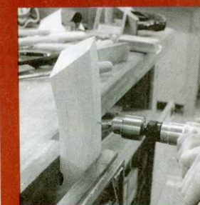
8 Drill a pilot hole first for the central bolt. Brian used a nut that screws into the top tier
