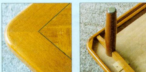
The lipping is held underneath by glue blocks at the corners
