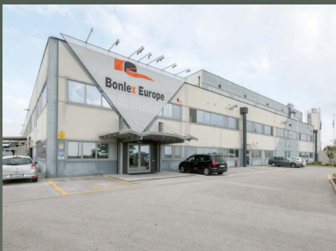
The brand new recycled PET line is one of four lines at Motta di Livenza.
