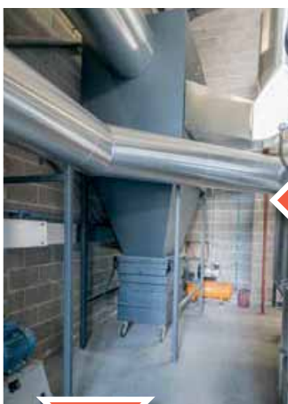
A multi cyclone that takes out the larger pieces of ash in the airflow.
