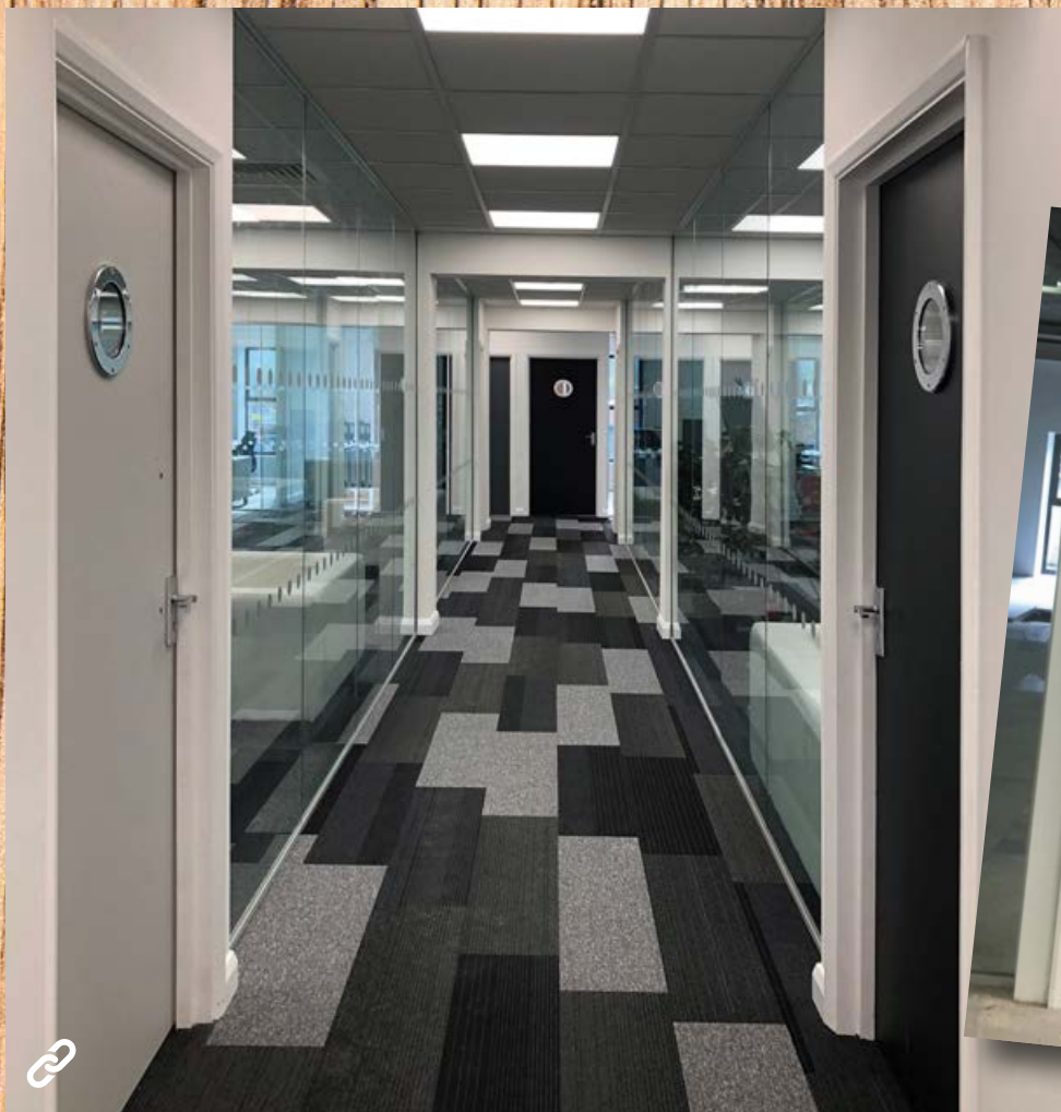
Background: EL194. Below: Door before. Left: Doors and space after refurbishment.
