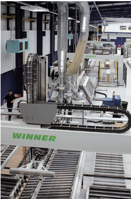
Above: A BiesseEdge Stream SB1 combination edgebander installed in a fully automated cell using RBO Winner loaders and unloaders.
