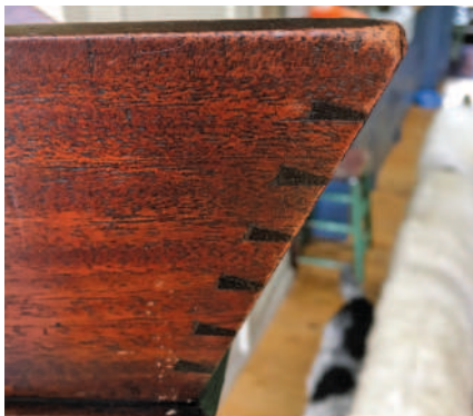
Faux dovetails – actually dovetail keys
