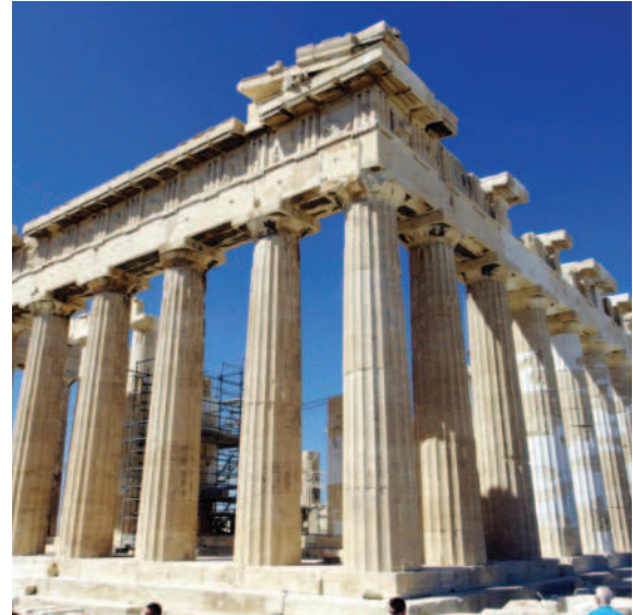
The columns of the Parthenon in Athens showing entasis
