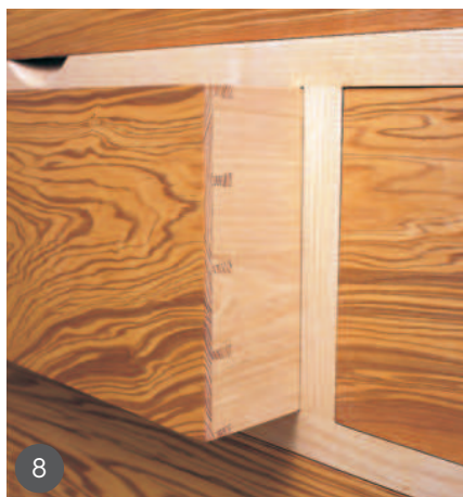
8 Traditionally lapped dovetails on the drawer fronts 9 Runners and kickers 10 Central runners and kickers
