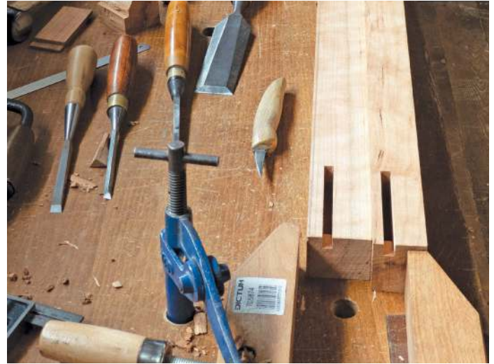
Working on the mitred mortises
