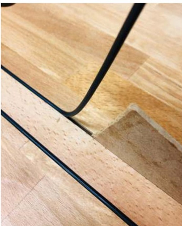
16. A 3.5mm rubber gasket was pushed into the 3mm shadow gap
