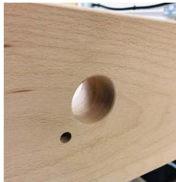
Clean straight holes are crucial for a good fit of the jaw
