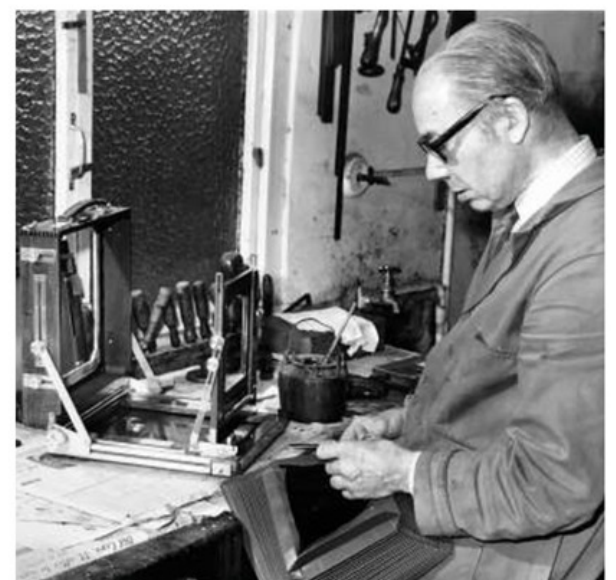
Fred attaching bellows to a rear standard
