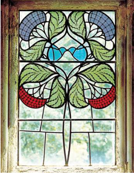
Stained glass panel from the Bedroom
