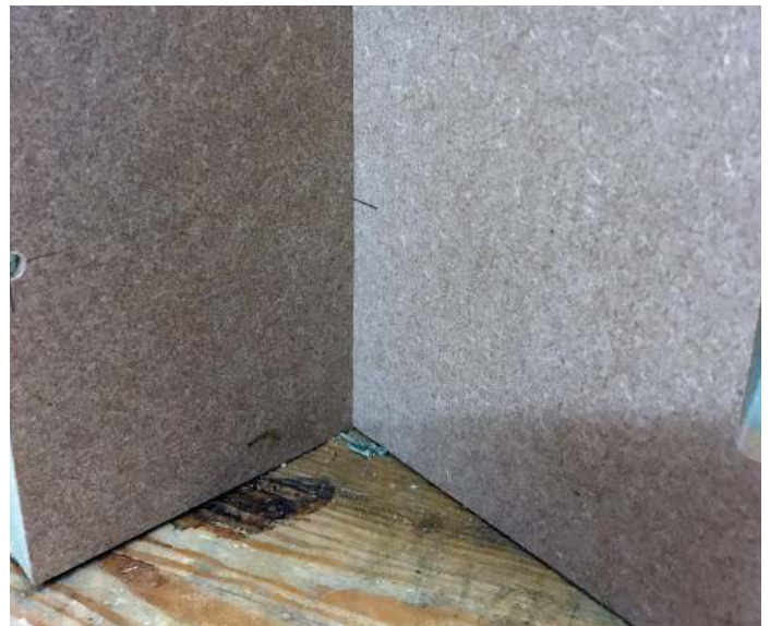
Domino and dowel screw are the strongest combination and pull up ridiculously tight
