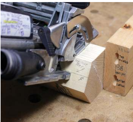
Line up the baseplate's milled flats to the centre line on the post, and lock up the fence height
