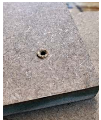
Delamination can occur on the exit side of the screw hole as well
