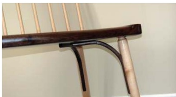
The braces mortised to the leg and screwed to the seat in this shaker bench
