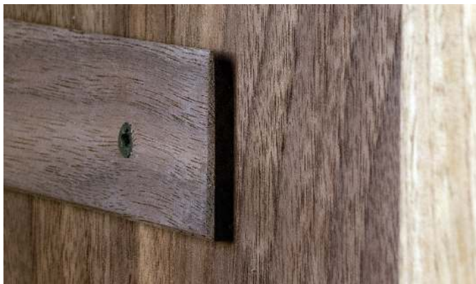
A dovetail shaped cleat holds the rack in place
