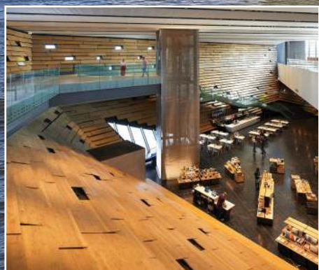
The stepped interior walls are lined with hanging oak-veneered panels, pierced by slot windows
