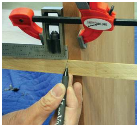
I used a story stick to figure out the dimensions for the cabinet back and opening
