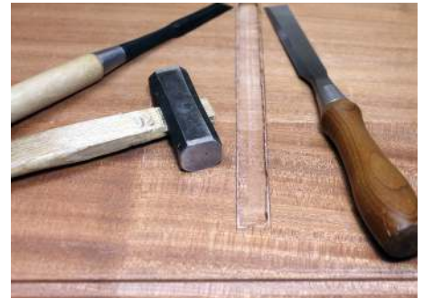
Careful chisel work produces first-class joinery fit for the centre divider
