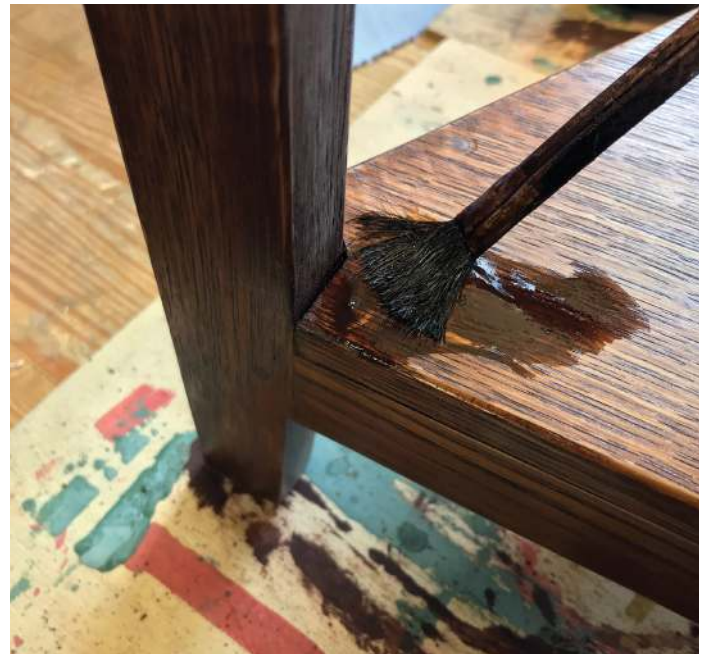
Apply the stipple all over and work into the corners and crevices
