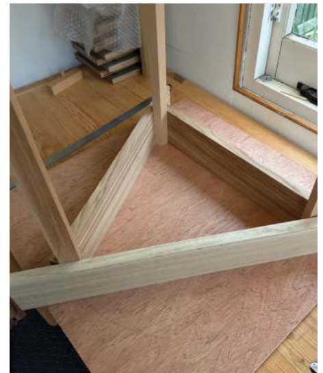
Checking the geometry of the components against the rod
