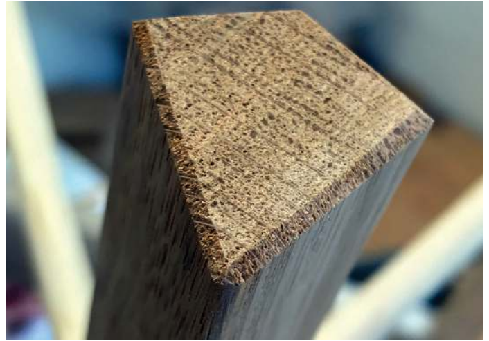
Chamfering the feet prevents the edges from splitting
