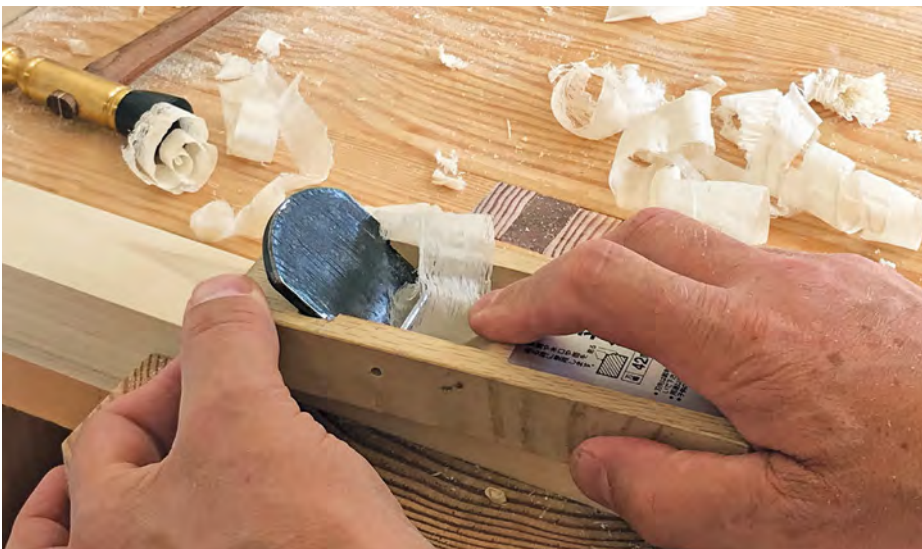
Flush up the joint afterwards
