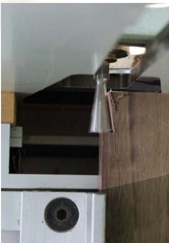
Cutting the half socket shoulder
