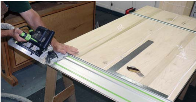
Cutting the mitres RIGHT: Cleaning up the mitres
