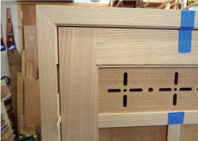
Set back chamfer detail used around doors and drawers
