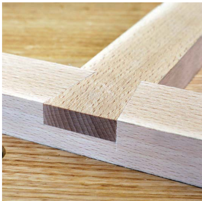
Dovetail halving joint
