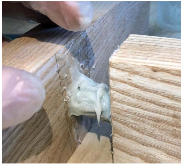
Ensure sufficient resin is applied to fill any voids
