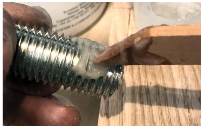
Apply the thicker resin mixture to the bar
