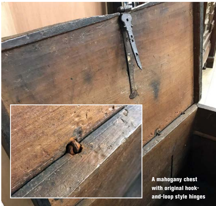
Waxed cranked hinge with penny rounds detail at the ends of the leaves INSET: Don't look for precision in strap hinges, you won't find it
