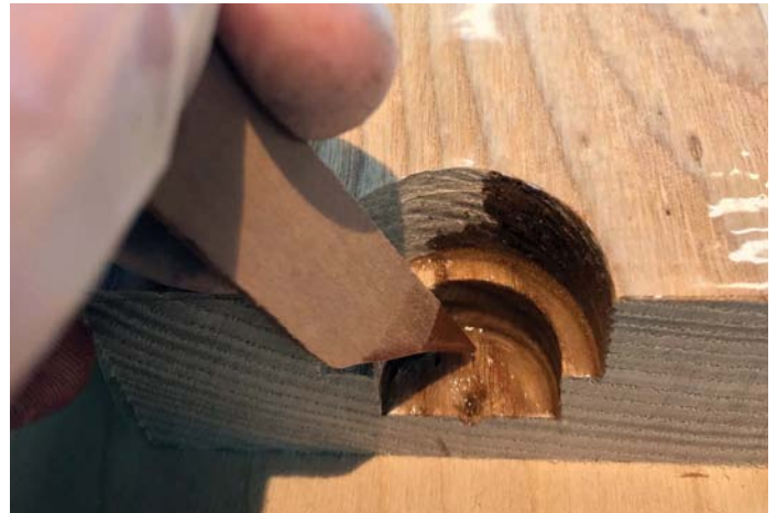
Use a basic resin to completely wet out the hole
