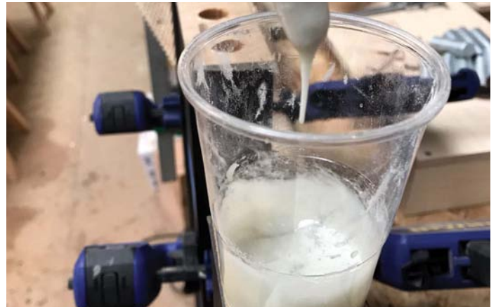
Add filler to the resin to bulk it out and strengthen the joint
