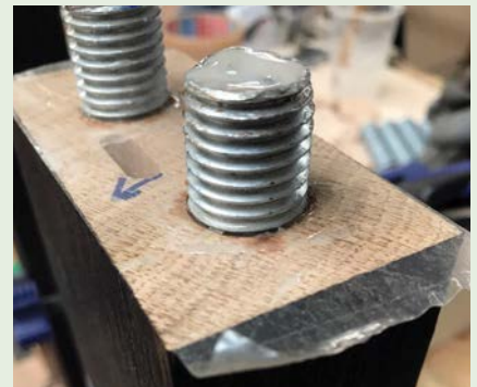
When the resin has cured the tape is removed
