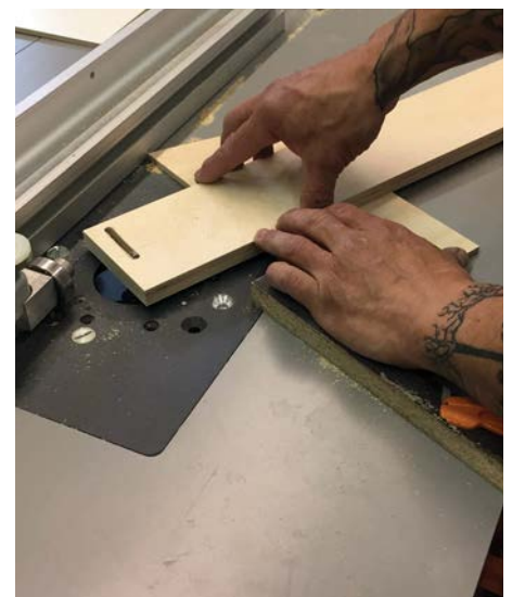
Place a packer beneath the fence piece
