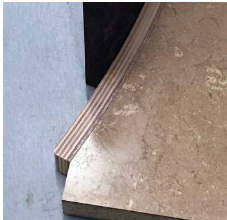
The particle board is faced with ply from the duplicate
