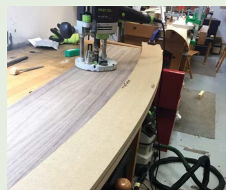
This 4.5m radius template was one of many ordered in from an external source
