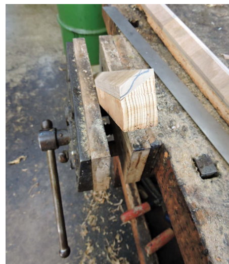
Sections of deal are chamfered before adding the show wood
