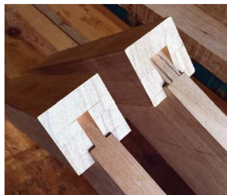
Housed tenon and housed sliding dovetail joinery options
