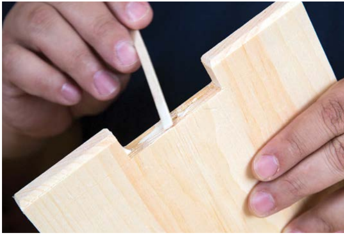
Apply glue to all the surfaces but don't go overboard. Cleaning up excess glue around joints is a pain
