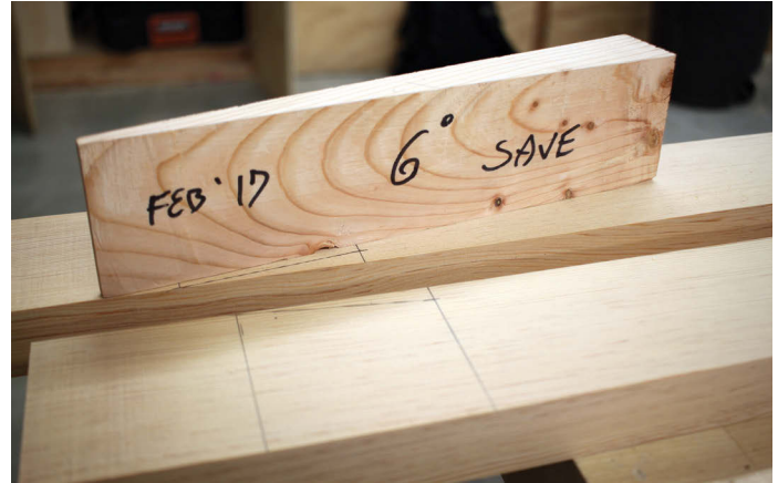
The corresponding shim is used to check progress
