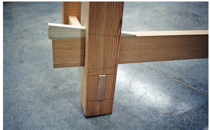
The tusk or wedge drives the joint together without the need for glue
