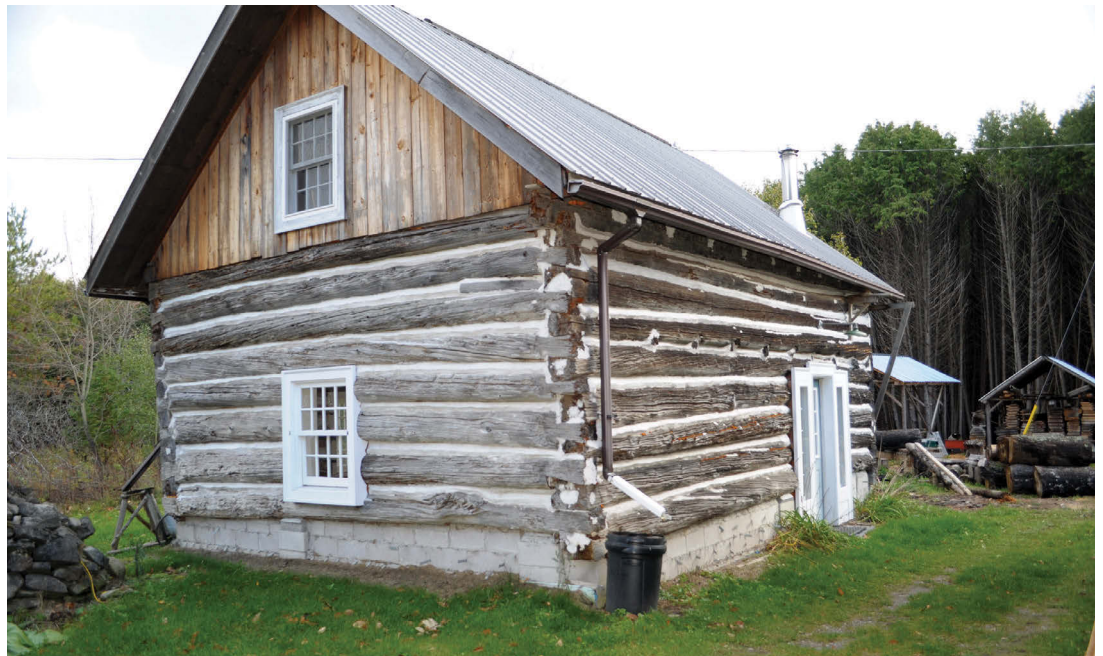
This log building on Michael's property has been renovated to include gallery space, a small design office and a loft apartment for an intern
