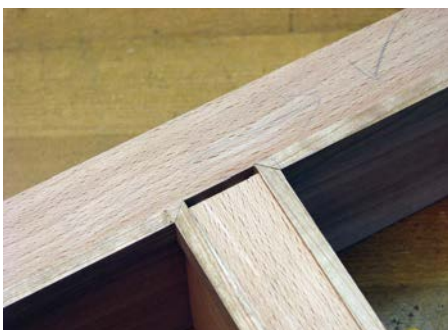
The gap in the through rabbet requires filling
